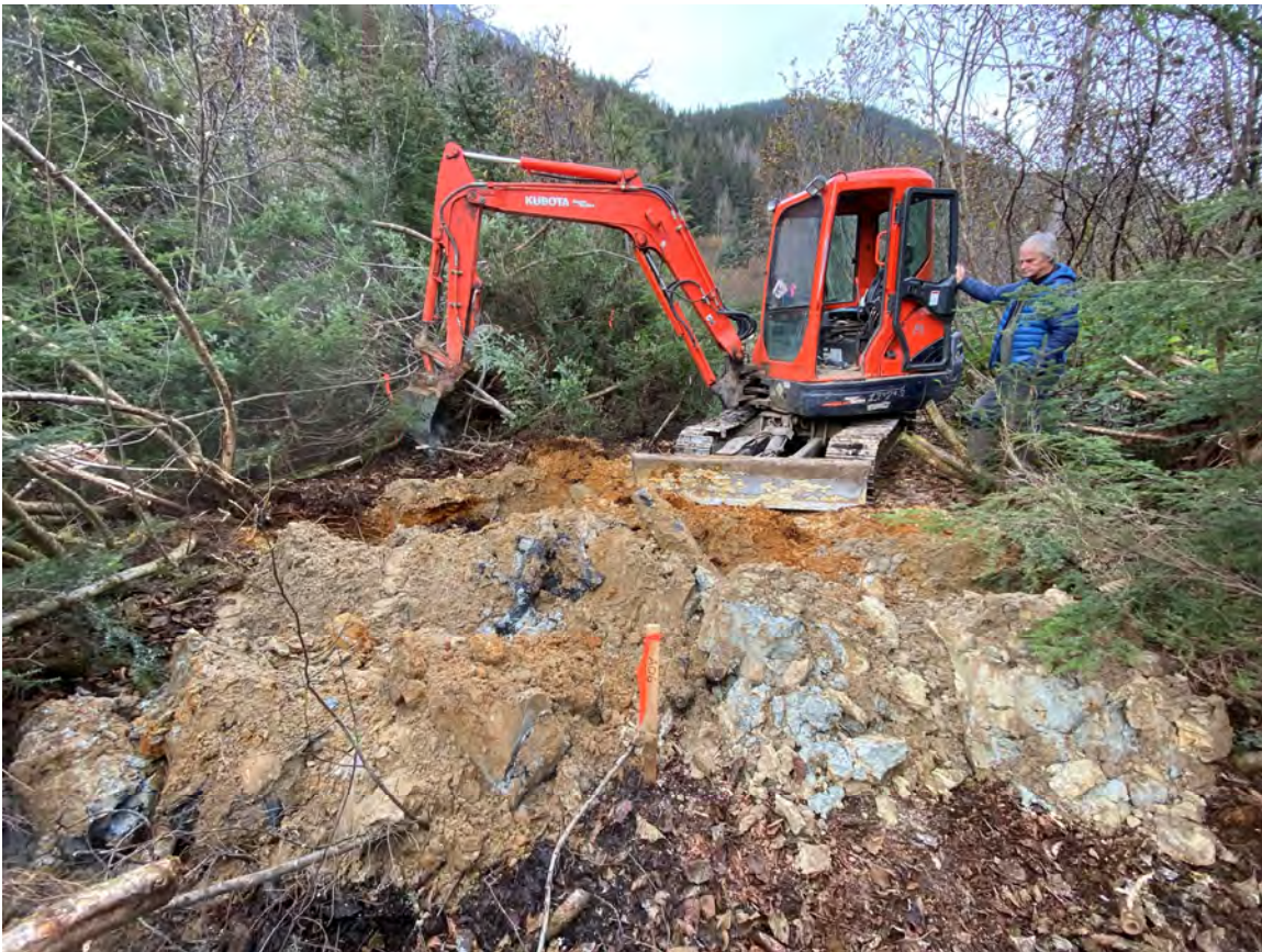
Figure 2: Example of test pit sample layout from A06 (top closest to excavator)
