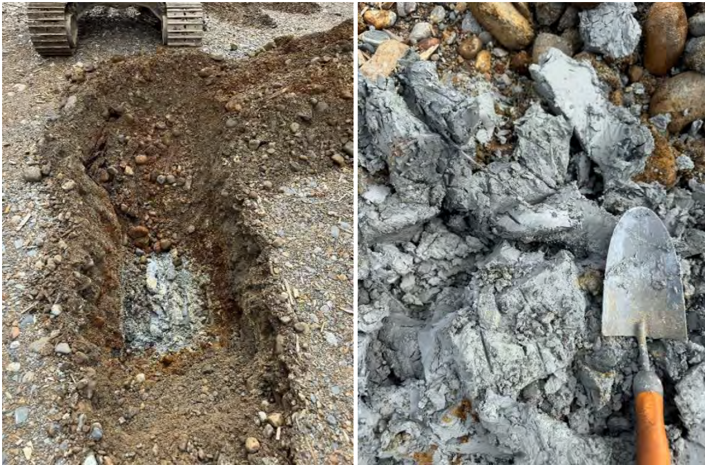
Photo 4 Test Pit LP2 - Lower Portal
