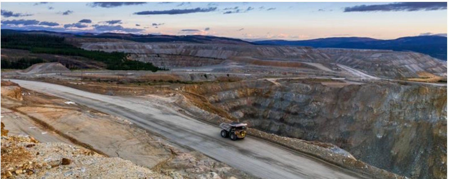
Figure 2-2: Existing HVC Mine Pits
