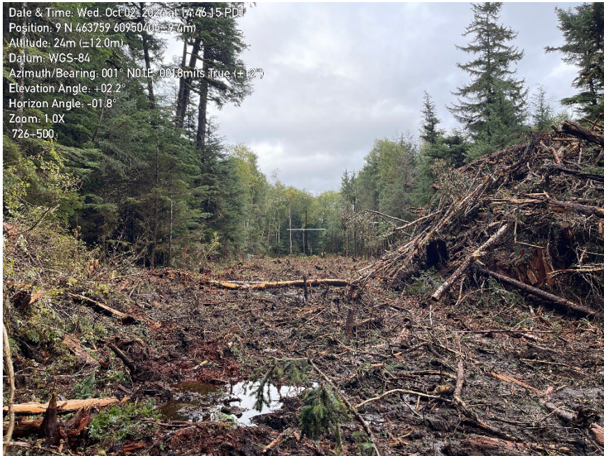
Photo 3. Cleared Project ROW at KP 726+500 in lowchain direction
