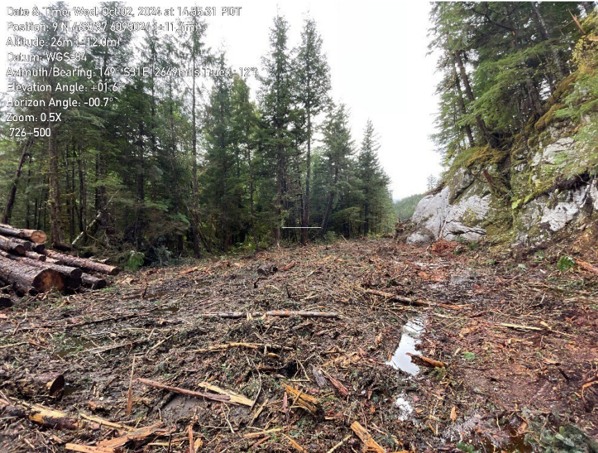
Photo 2. Cleared Project ROW at KP 726+500 in highchain direction.
