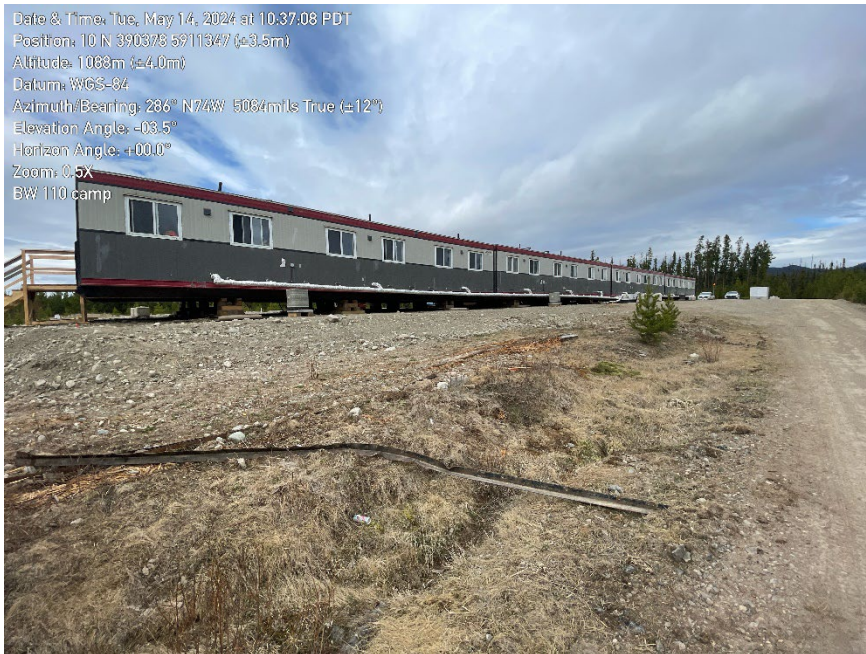
Photo 1. Camp, East side of main wing.
