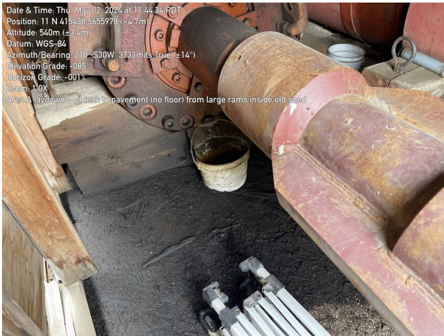
Photo 5: Large hydraulic ram leaking oil to ground. The shed that it’s in has no floor.
