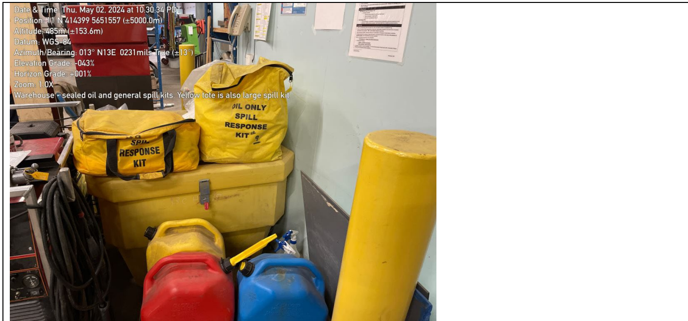
Photo 4: Sealed spill kits in the warehouse. At least one of them is "oil only". The large, yellow plastic tote is a spill kit as well.
