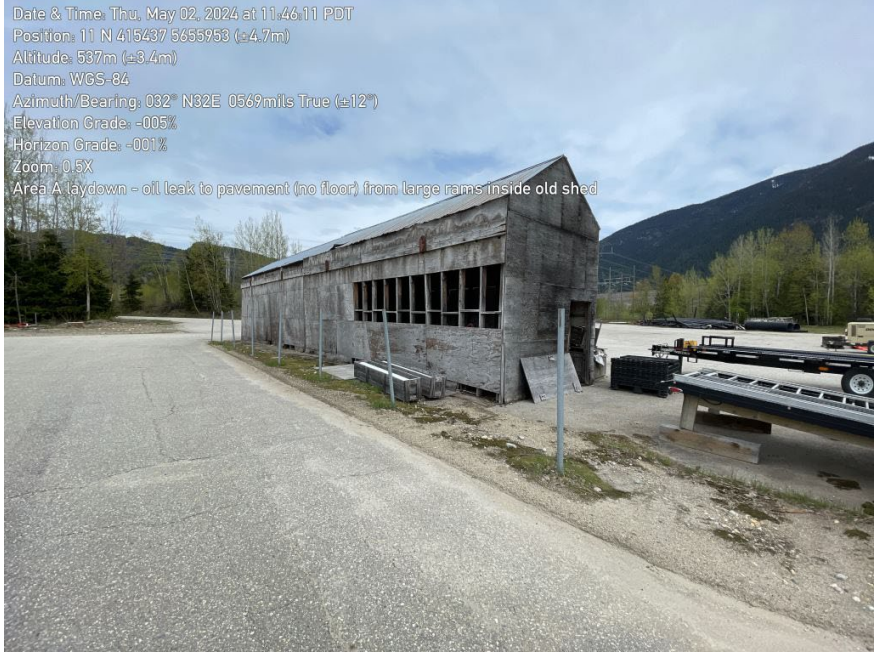
Photo 6: The shed that contains the hydraulic ram.
