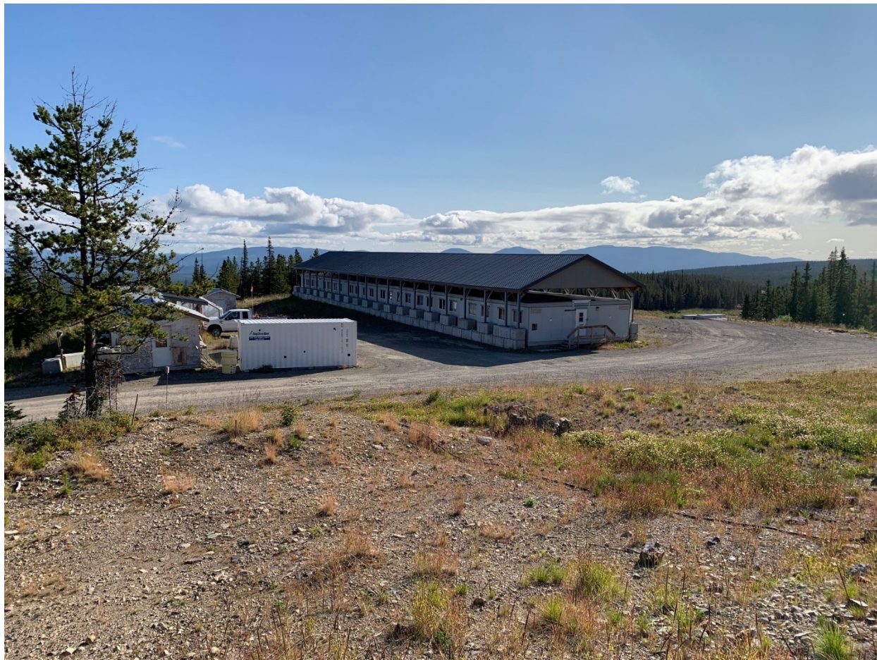
Photo 27: Camp Trailers (Area 11)
