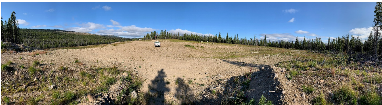
Photo 4: Sewage Discharge Field (Area 1)
