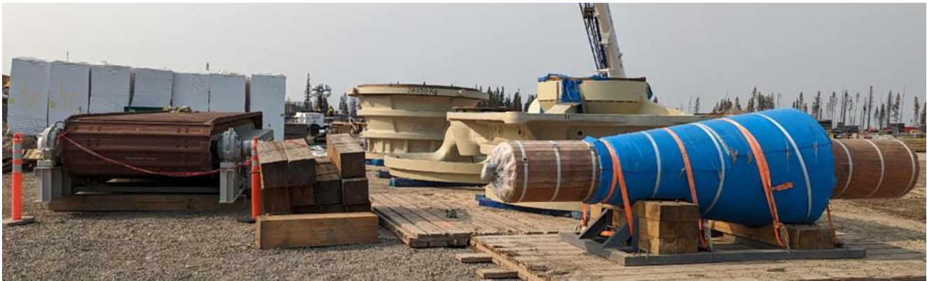
Apron feeder and primary gyratory crusher
