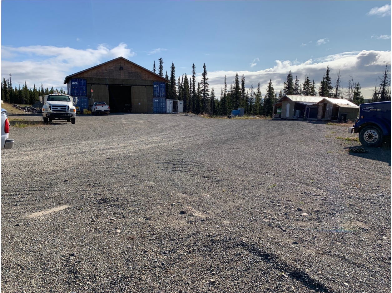
Photo 18: Maintenance Facility, Cold Storage, Laydown Area (Area 9)
