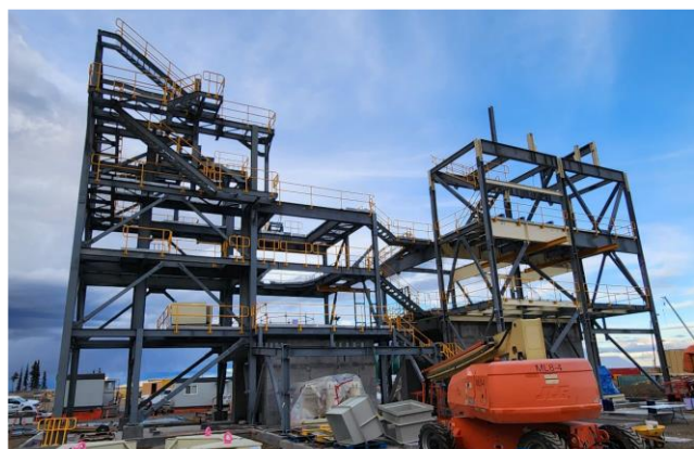
Secondary and tertiary crusher structural steel – October
