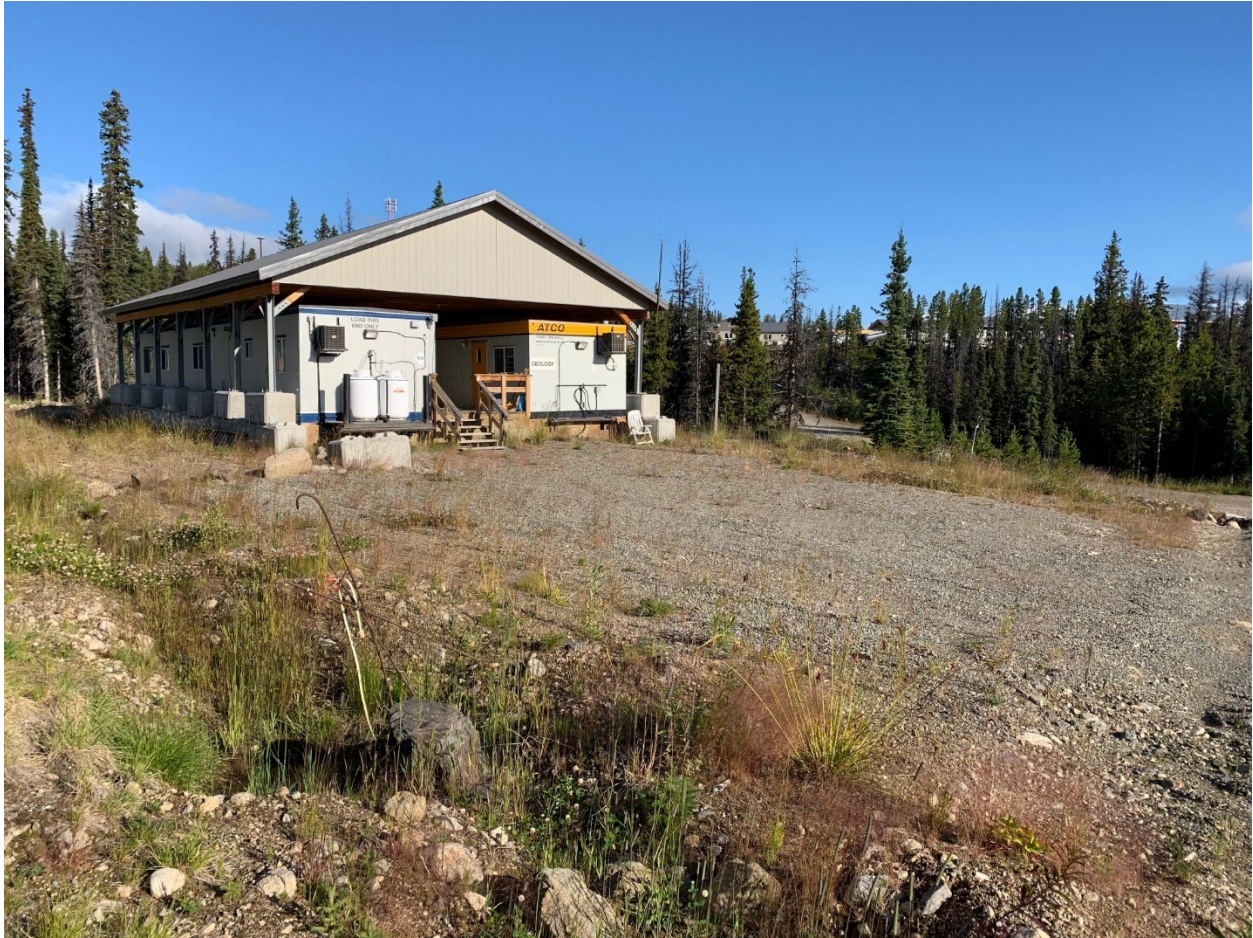
Photo 15: Geology Office (Area 7)
