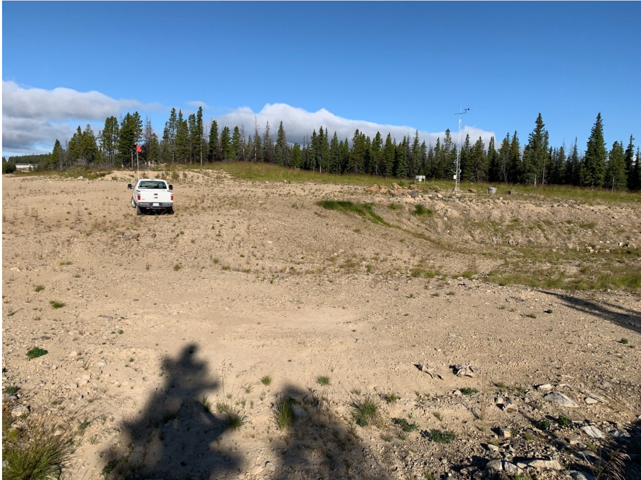
Photo 3: Sewage Discharge Field (Area 1)
