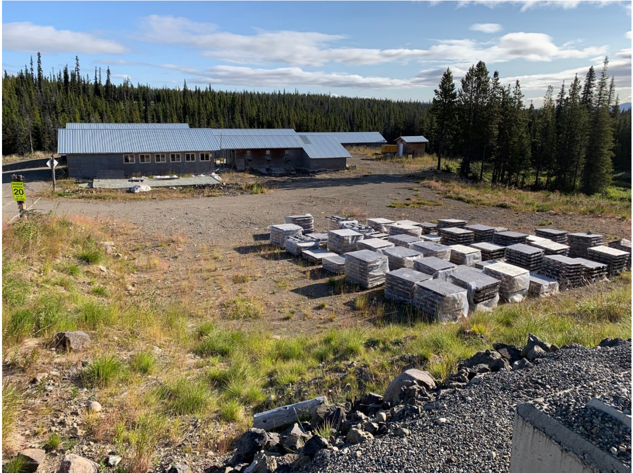
Photo 12: Laydown and Incinerator (Area 4)
