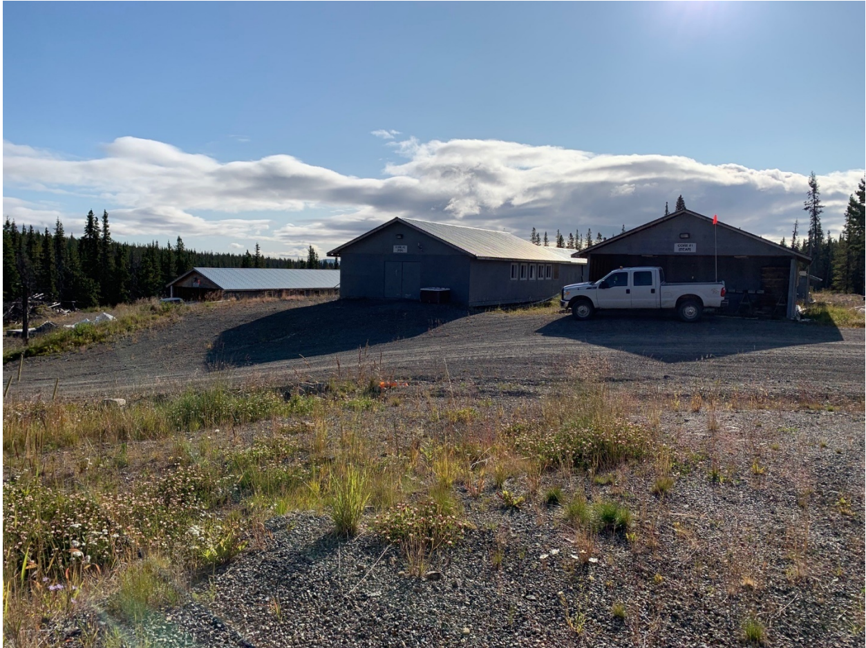
Photo 14: Core Processing Facilities (Area 5)
