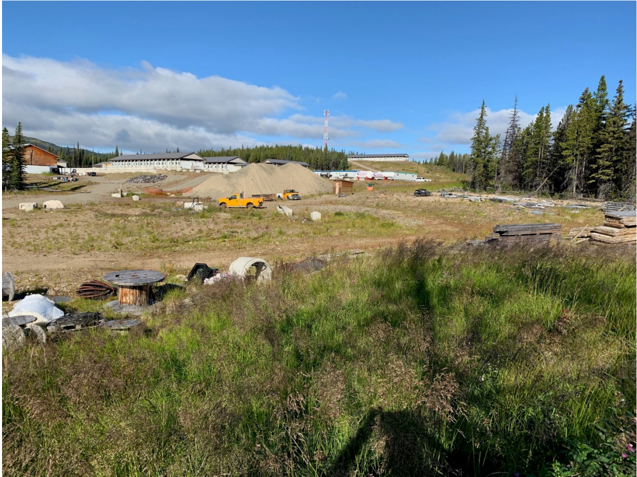
Photo 16: Sewage Treatment and Laydown Area (Area 8)
