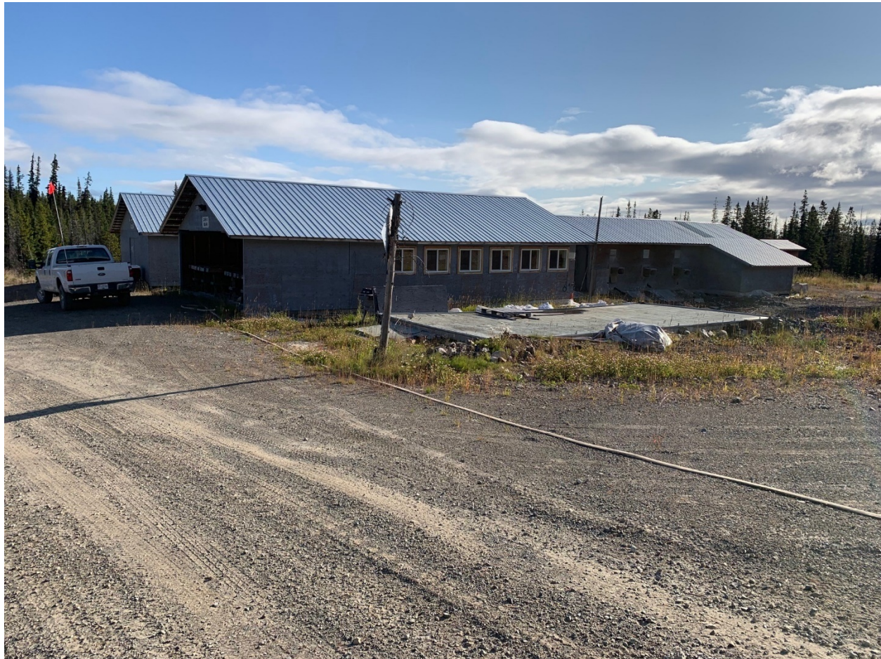
Photo 13: Core Processing Facilities (Area 5)
