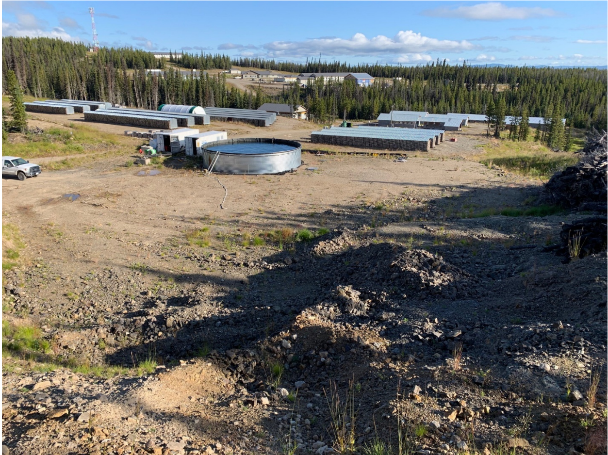
Photo 11: Laydown and Incinerator Area (Area 4)
