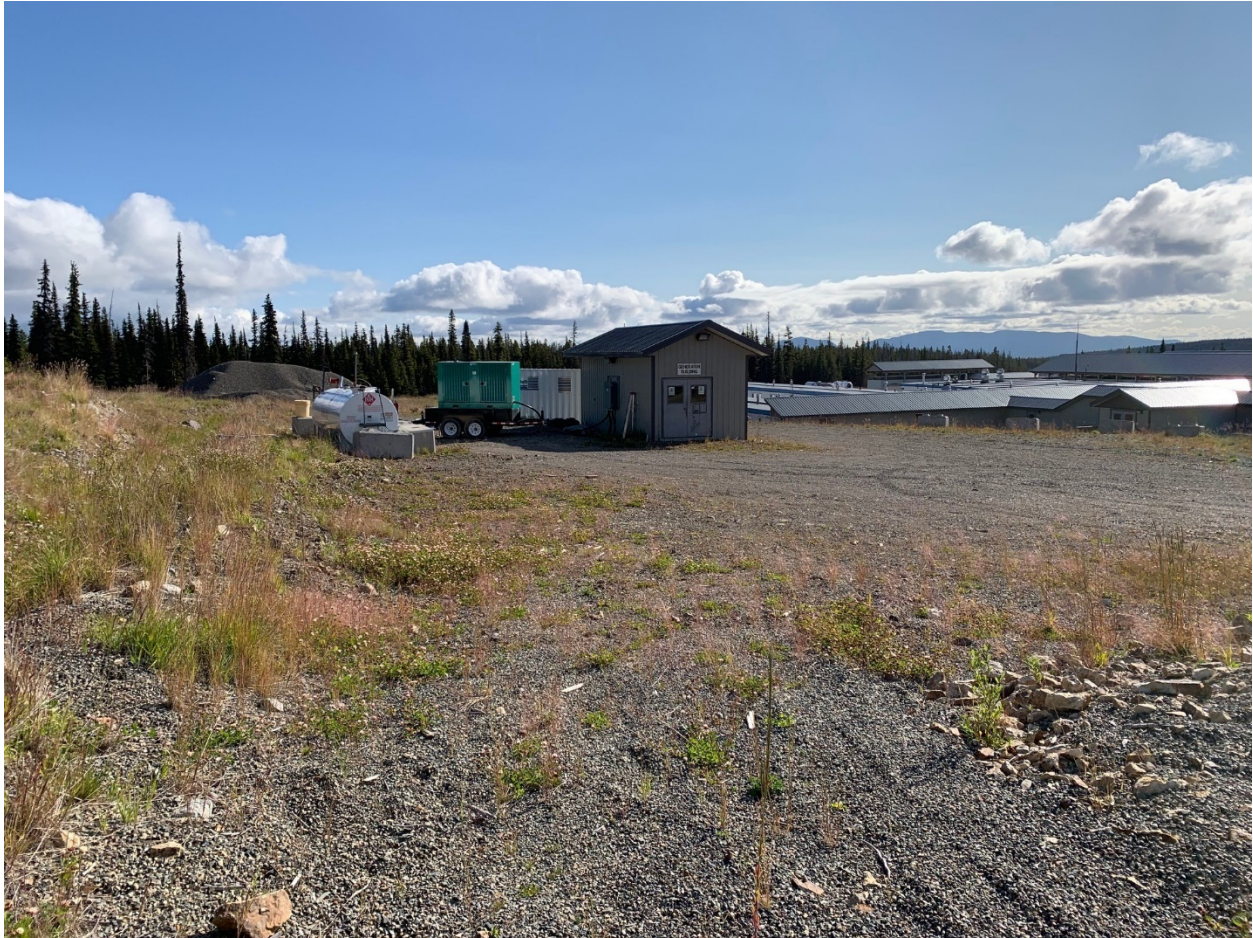
Photo 19: Generator Building (Area 10)
