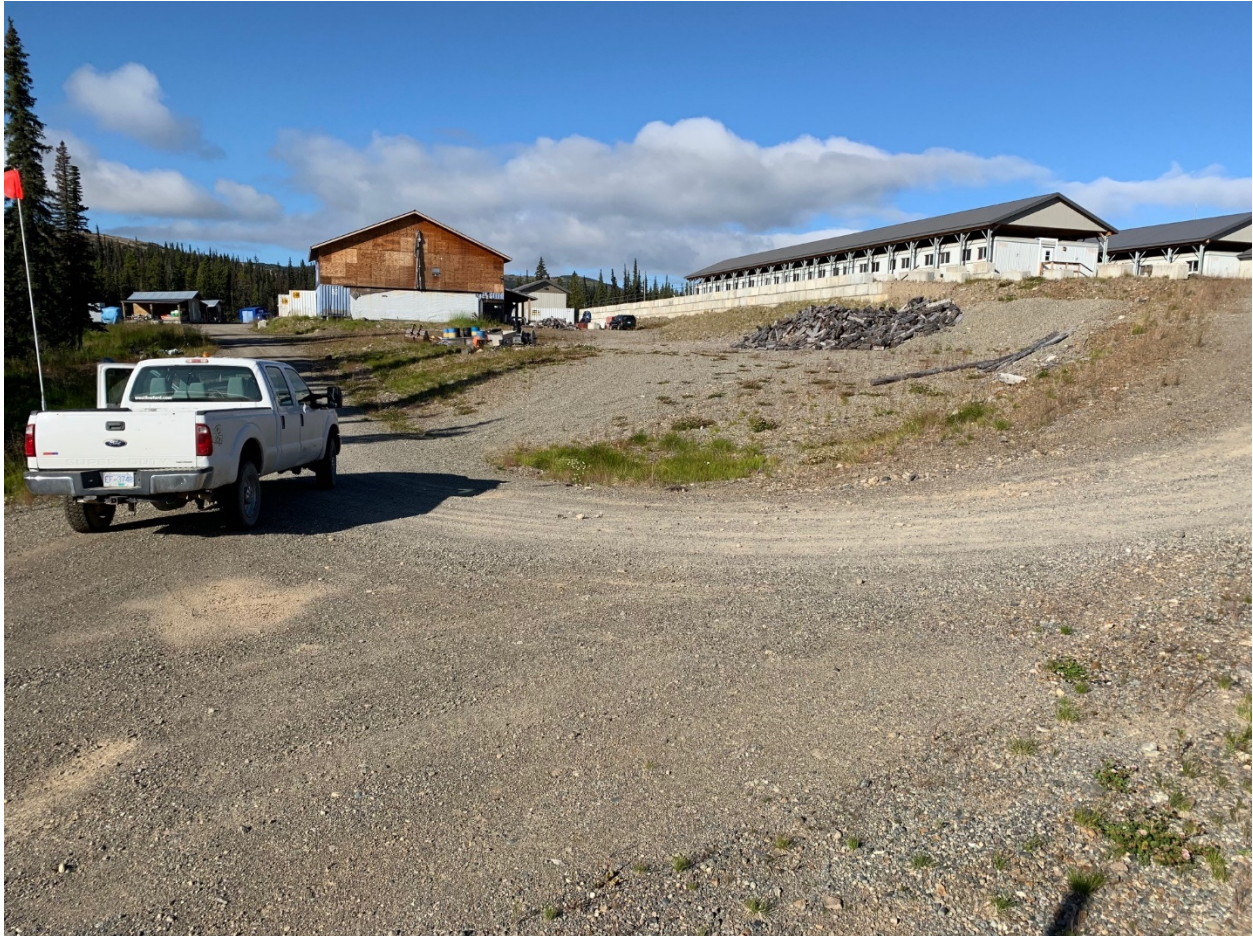
Photo 17: Maintenance Facility, Cold Storage, Laydown Area (Area 9)
