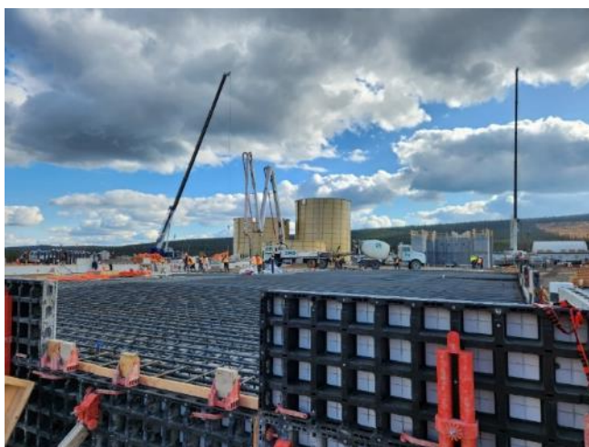
Reagents building civil works – September
