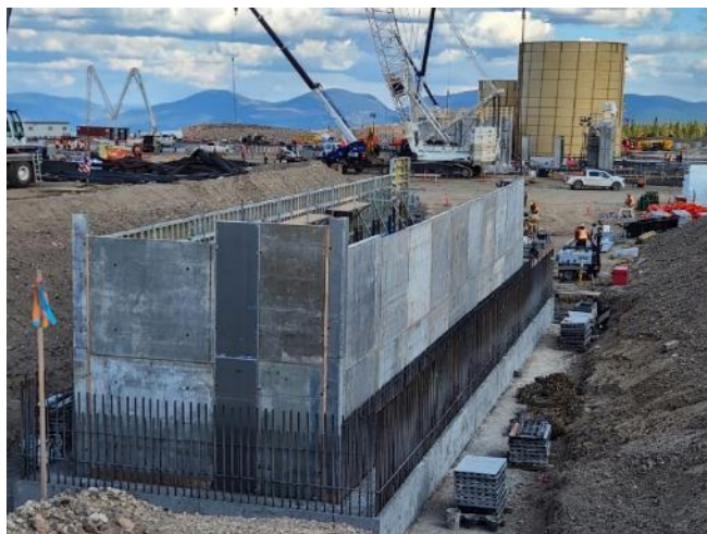
Reclaim tunnel – civil works – September
