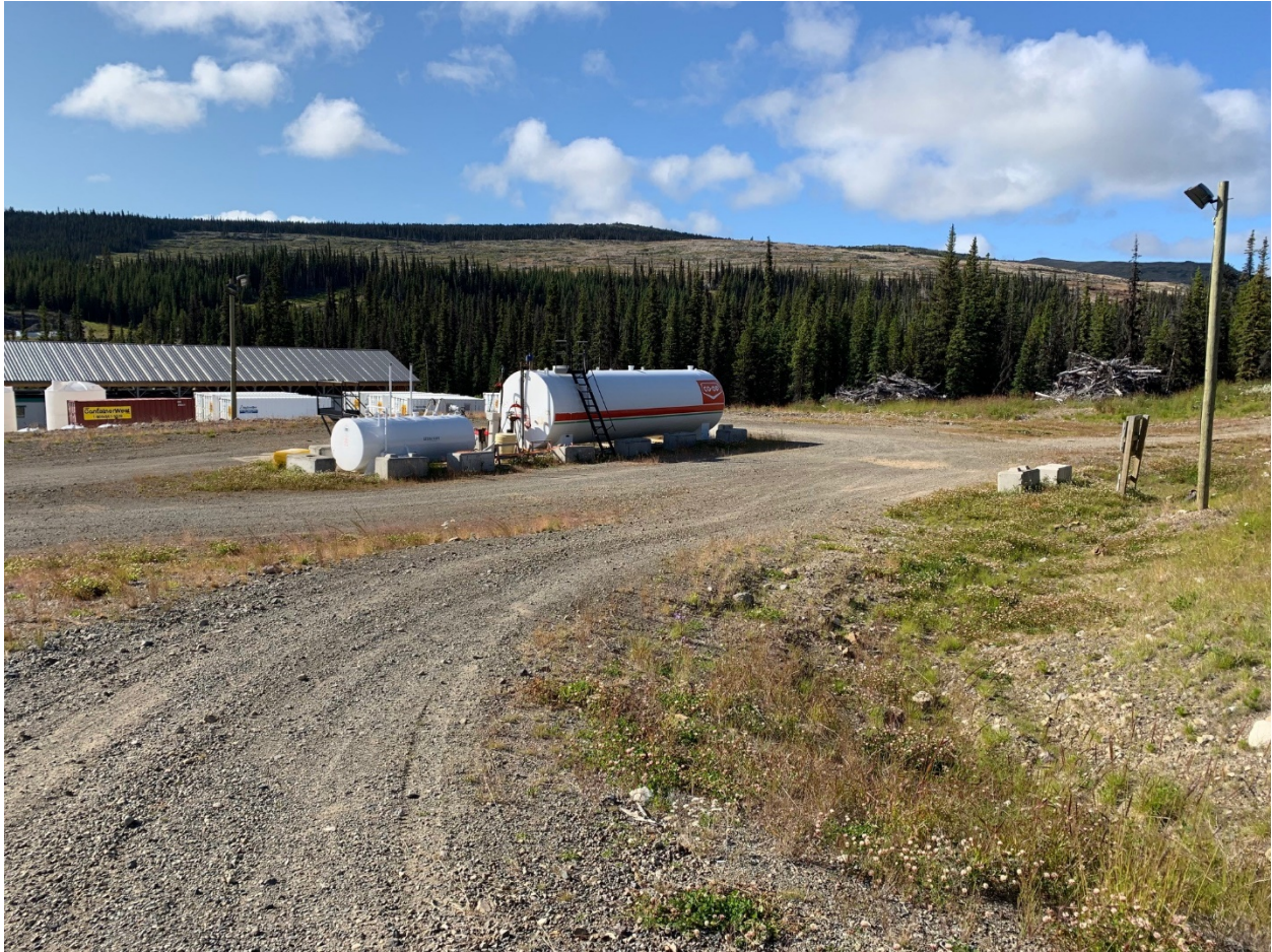
Photo 29: Main Fuel Island (Area 13)
