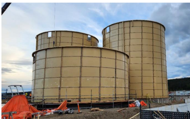
CIL tank construction – October
