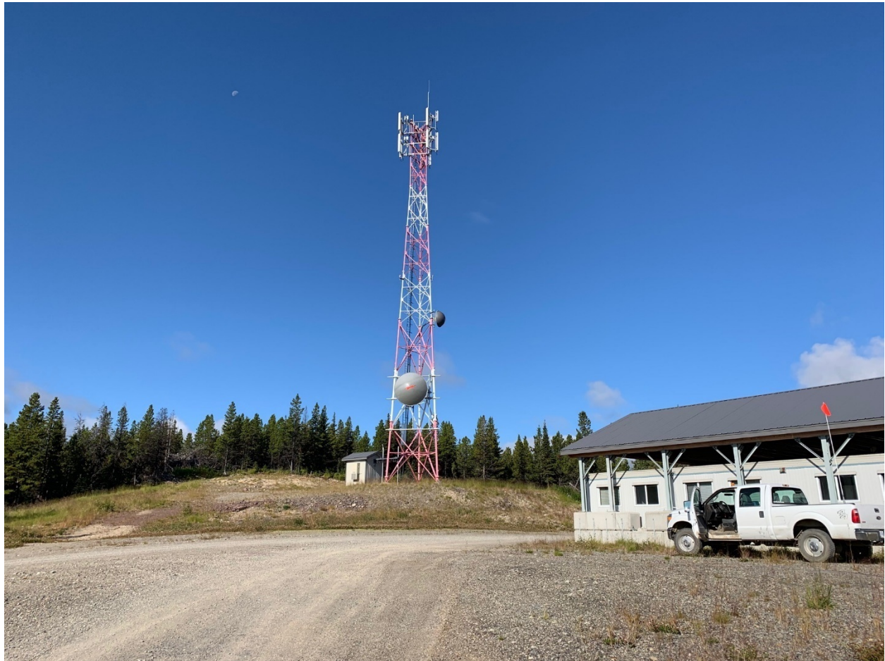
Photo 30: Communications Tower (Area 14)
