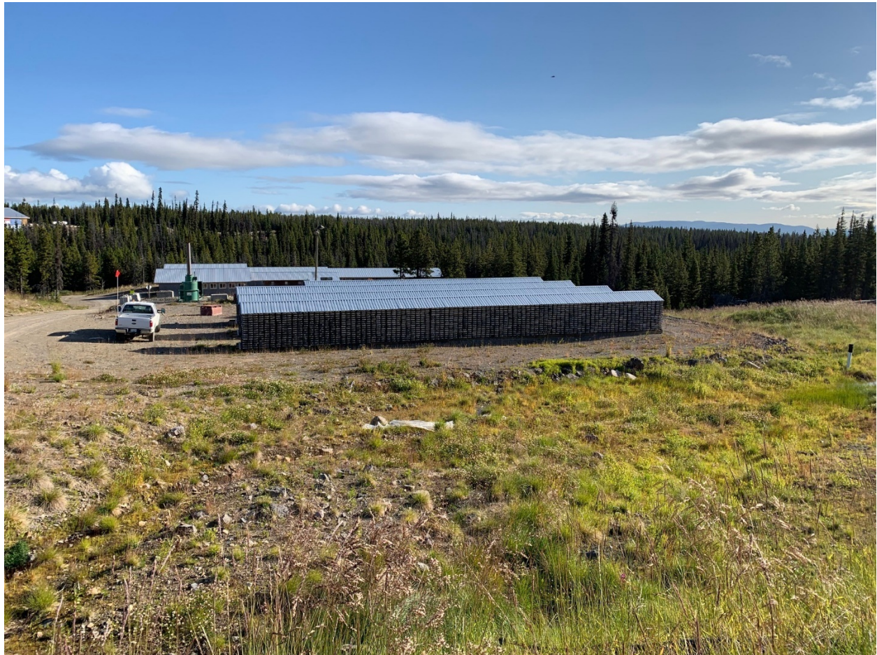
Photo 10: Laydown and Incinerator Area (Area 4)
