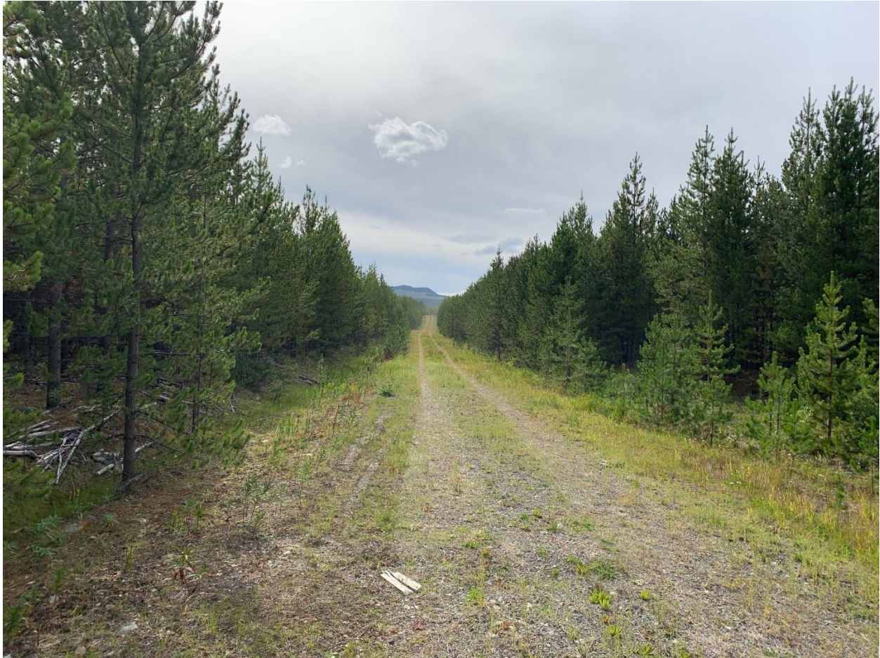
Photo 2: Airstrip Access Road Near Mine Access Road
