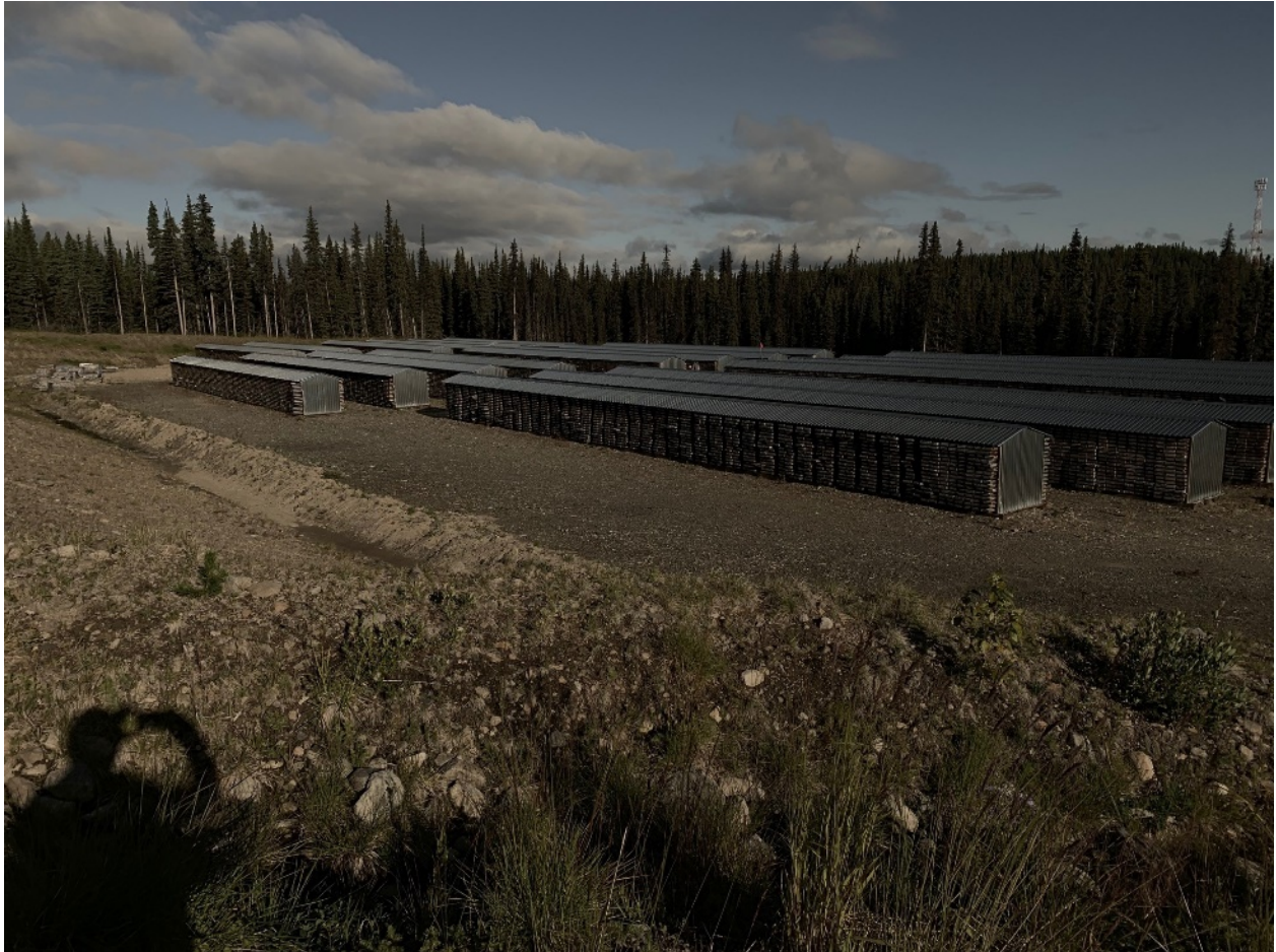
Photo 9: West Core Storage Area (Area 3)
