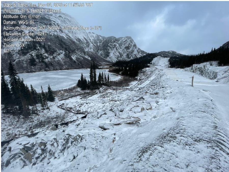
Photo 11. KP 141+100 approximately. Perimeter controls and cover management per the WEP.
