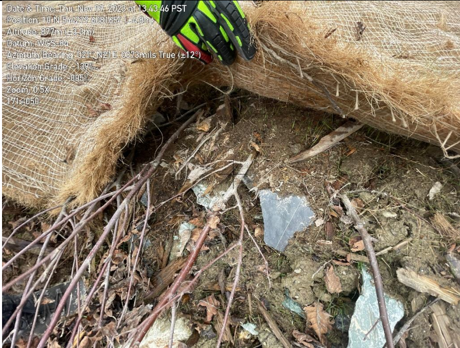
Photo 9. Close-up of willow staking at the watercourse crossing at KP 171+050.
