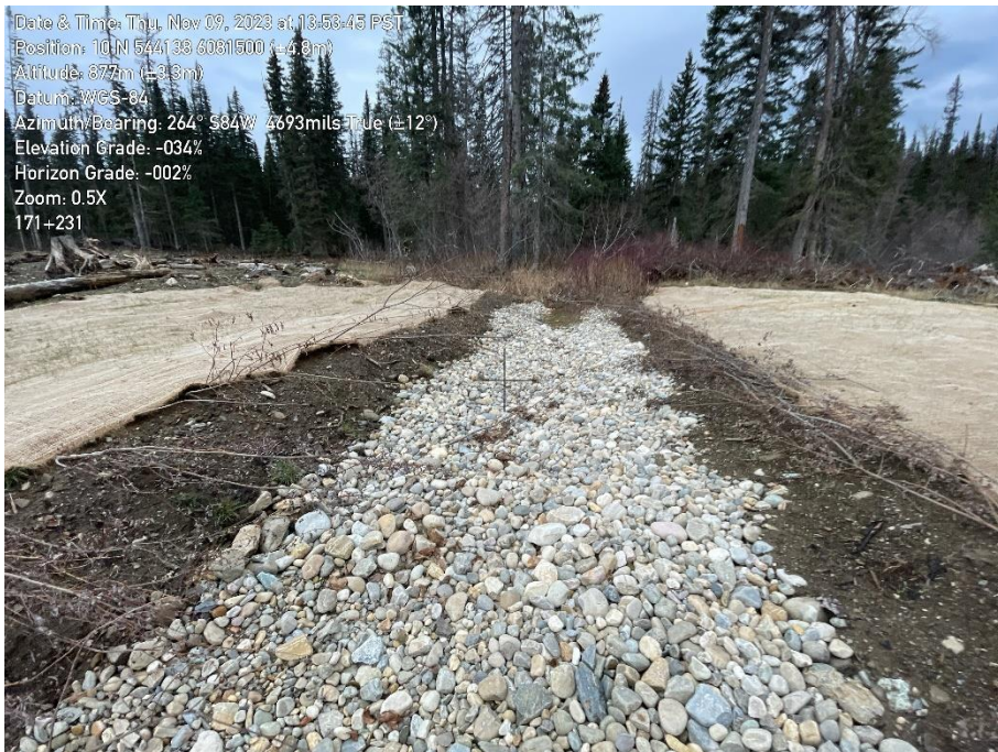
Photo 4. Watercourse number J234.99 looking upstream to downstream – mid crossing channel.
