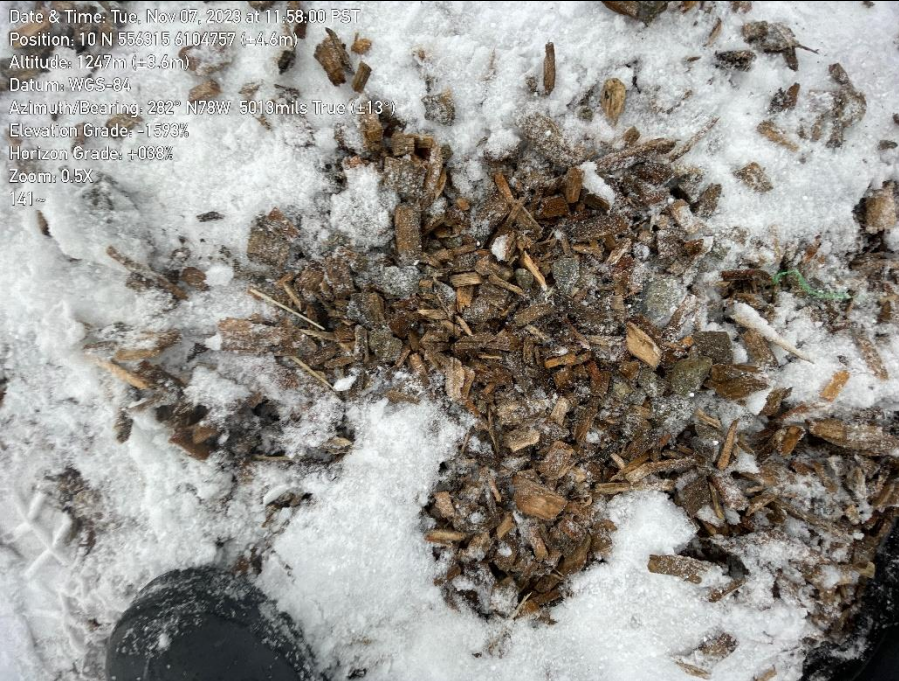
Photo 12. KP141+100 approximately. Close up of wood mulch used as cover management.
