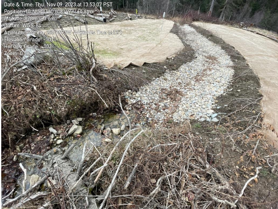
Photo 3. Watercourse number J234.99 looking upstream to downstream - overview.
