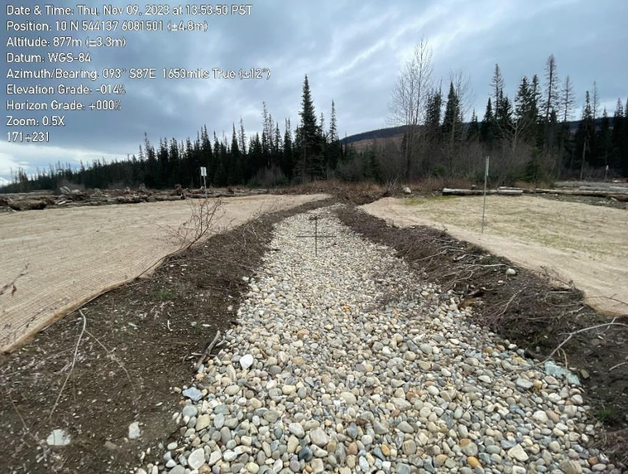
Photo 5. Watercourse number J234.99 looking downstream to upstream.
