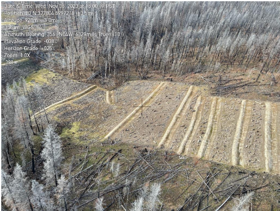
Photo 14. Overview of KP 381 as seen from the air on November 8, 2023. Final clean-up completed.
