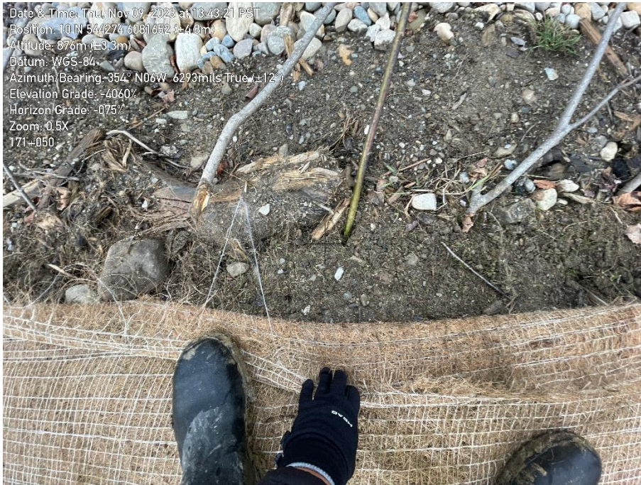
Photo 8. Close-up of willow staking at the watercourse crossing at KP 171+050.
