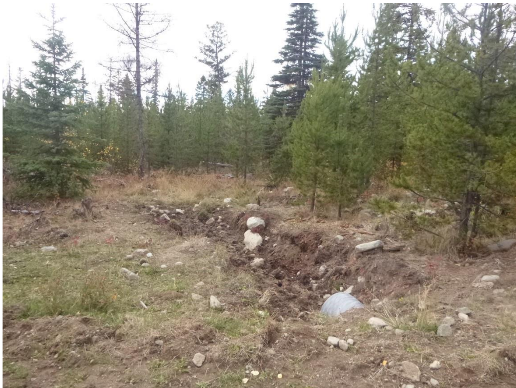
Photograph 4. Culvert across an access road in the Project area. Culvert was dry at the time of the site visit (September 29, 2021).
