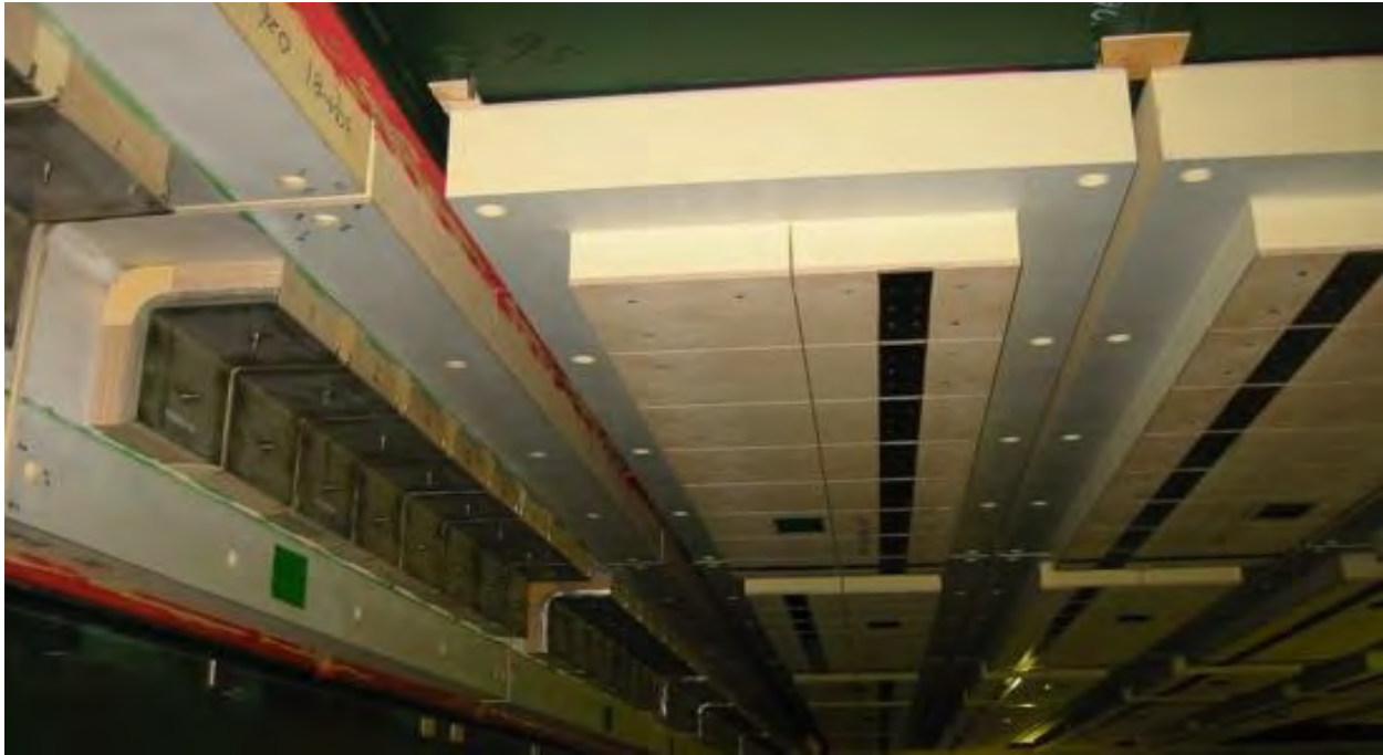
Figure 6 – GTT No. 96 Invar primary and secondary barrier
