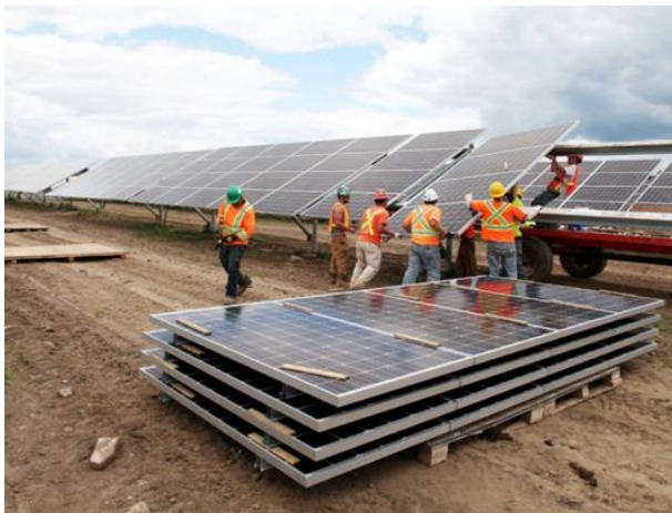
Typical installation of PV modules.
