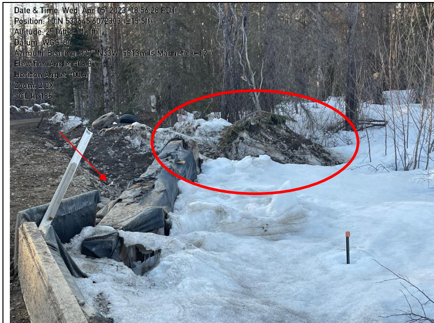
Photo 8: Dirty melting snow pile next to watercourse and ditch directed towards watercourse.
