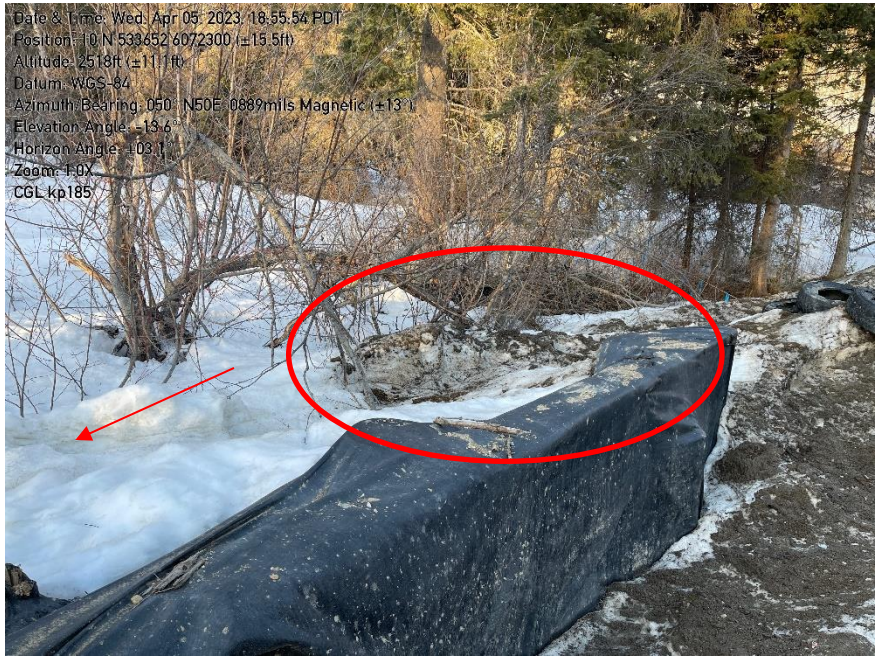
Photo 7: Dirty melting snow piled next to bridge crossing.
