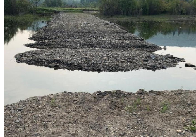
1 - Temporary Causeway for Reservoir Clearing (causeway example)
