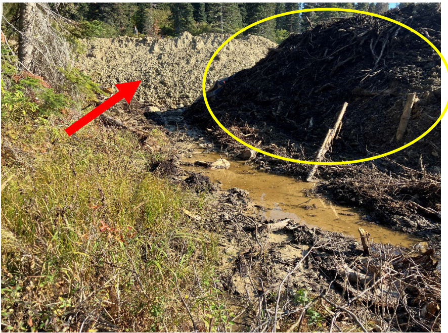
Photo 3: Approximately KP148+550. Soil and stripping piles not shown in WEP. No observation of sediment fence or woody debris berms specified in the WEP for sediment erosion control between sediment laden water and wetland WL0733. No observation of sediment erosion control between soil pile and sediment laden water.
