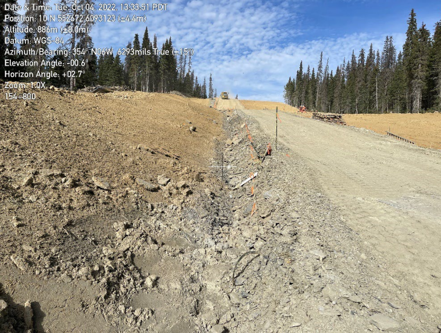
Photo 2: KP154+800. Rock lined ditch not complete, terminates into spoil pile down slope near Environmentally Sensitive Receptors (ESRs), Anzac River below.
