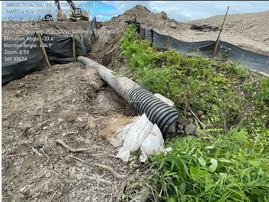
Photo 17. Culvert directing S6 watercourse 33C2A under the ROW at 369+280 non-functional as inlet was observed to be six inches above ground level.
