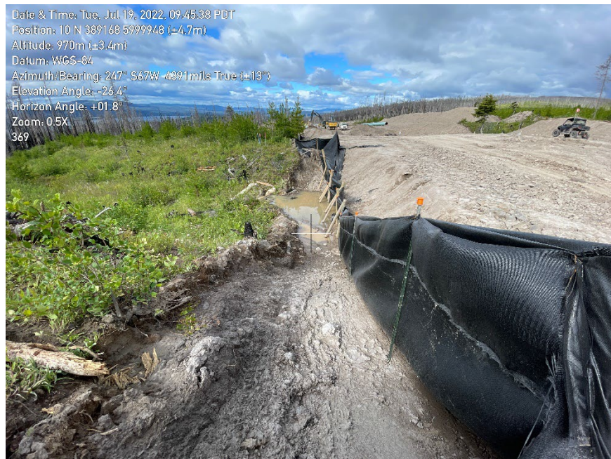
Photo 16. Erosion rills beyond gap in sediment fence on the downstream side of watercourse 32C2A (NCD) at KP369+200, with pooled sediment-laden water at the culvert under the ROW.
