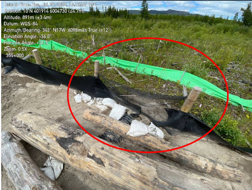
Photo 14. Gap in sediment fence between ROW and wetland WL-11401 (ESIW) at KP355+110.
