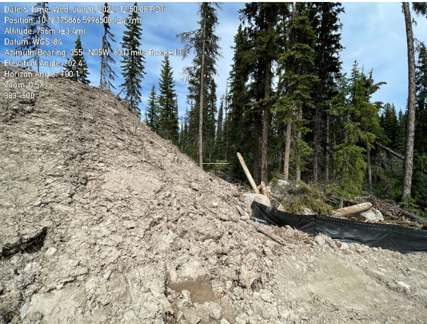
Photo 12. Spoil pile without erosion control measures adjacent to wetland WL-0684 (ESIW) at KP383+500.
