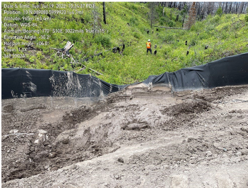
Photo 18. Minimal repairs to bulging and previously overtopped sediment fence at S6 watercourse 33C2A at KP369+295.
