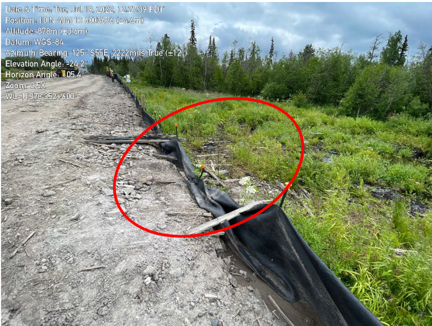
Photo 13. Collapsed sediment fence between travel lane and wetland WL-11378 (ESIW) at KP352+620.
