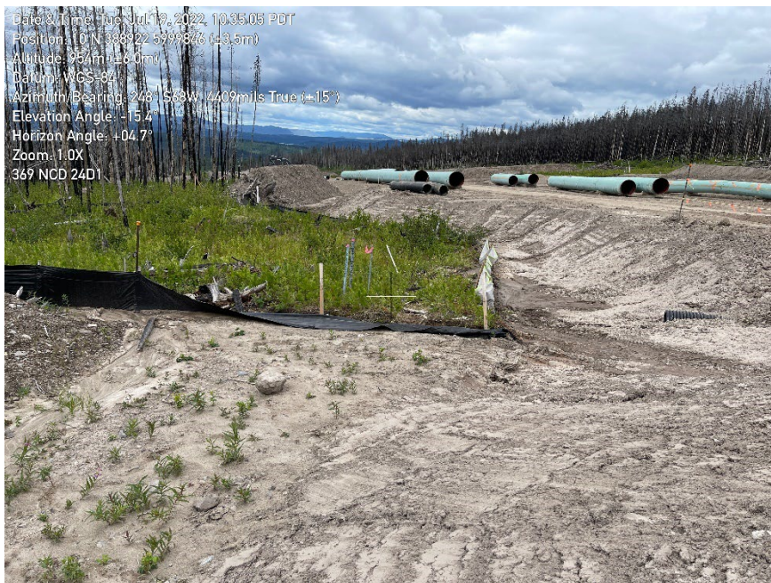
Photo 20. Non-functional sediment fence laying on the ground at watercourse 24D1 (NCD) crossing at KP369+480.
