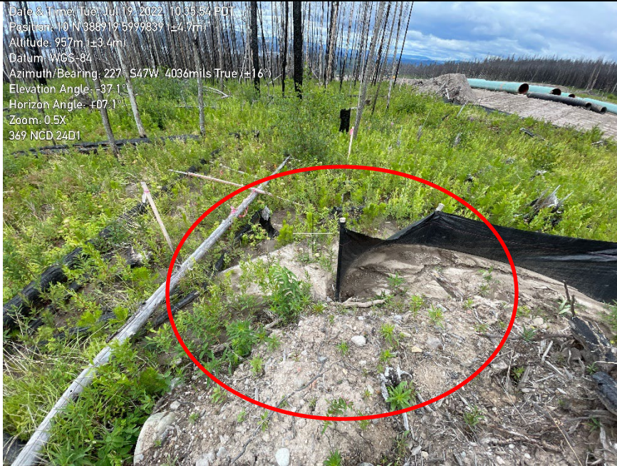
Photo 21. Evidence of sediment-laden water flowing around edge of sediment fence at watercourse 24D1 (NCD) crossing at KP369+480.
