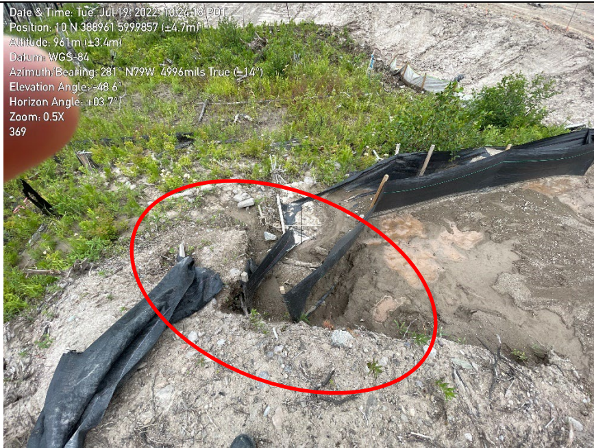
Photo 19. Newly installed sediment fence at watercourse 34C2A (NCD) at KP369+440 with gap at edge that will allow water to bypass.
