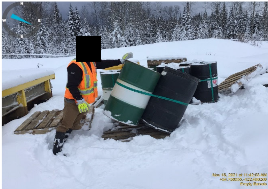
Photo 4: Parsnip MUS - The bulk chemical liquids stored without secondary containment were empty. The barrels identified in IR2021-027 Photo 29 and Photo 36 are now stored on a secondary container tray and the barrels have been covered with a tarp to prevent rain and snow from collecting in the tray (Photo 6).
