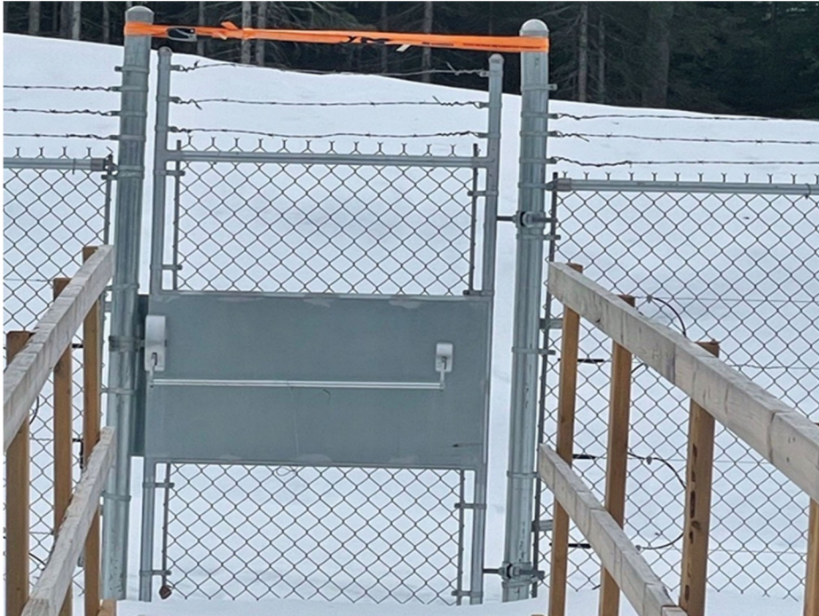
Photo 21: Headwall MUS man-gates with latches installed.
