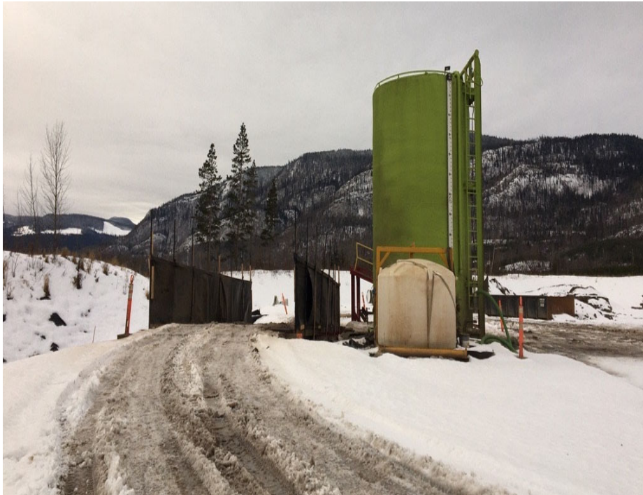
Photo 19: Sukunka Laydown 12 - Geotextile walls added to wash station.
