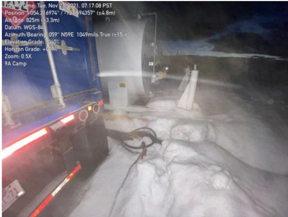
Photo 16: MUS 9A fuel island - secondary containment covered by recent snowfall
