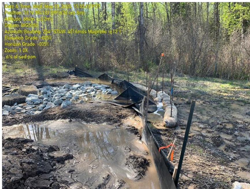
Photo 2: Failing ESC measures at boundary of Lejac MUS; ineffective in mitigating the turbid water discharge through active pumping.
