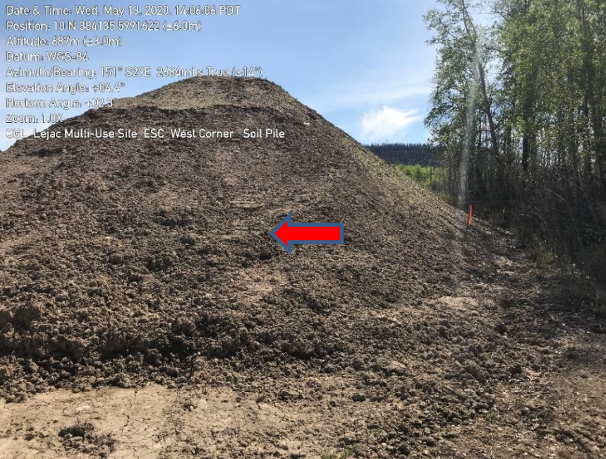
Photo 6: Soil Stockpile with no silt fence installed along base of slope, no evidence of seeding. Sluffing of soils depicted.
