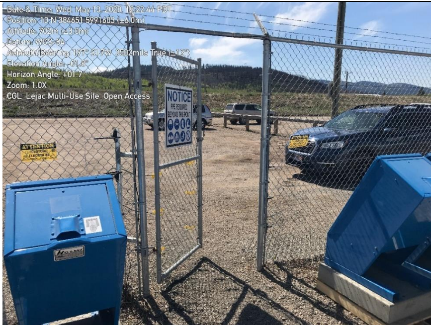
Photo 10: Access gate without functioning "self close" mechanism.
