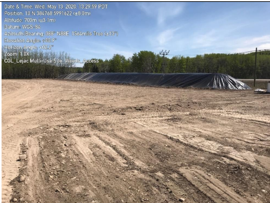
Photo 22: Area B, Covered topsoil stockpile to control noxious weeds.
