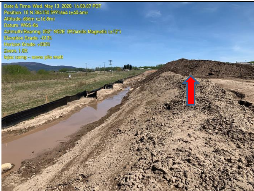
Photo 8: Snow stockpile depicted in background, ESC measures of wattle and silt fencing.
