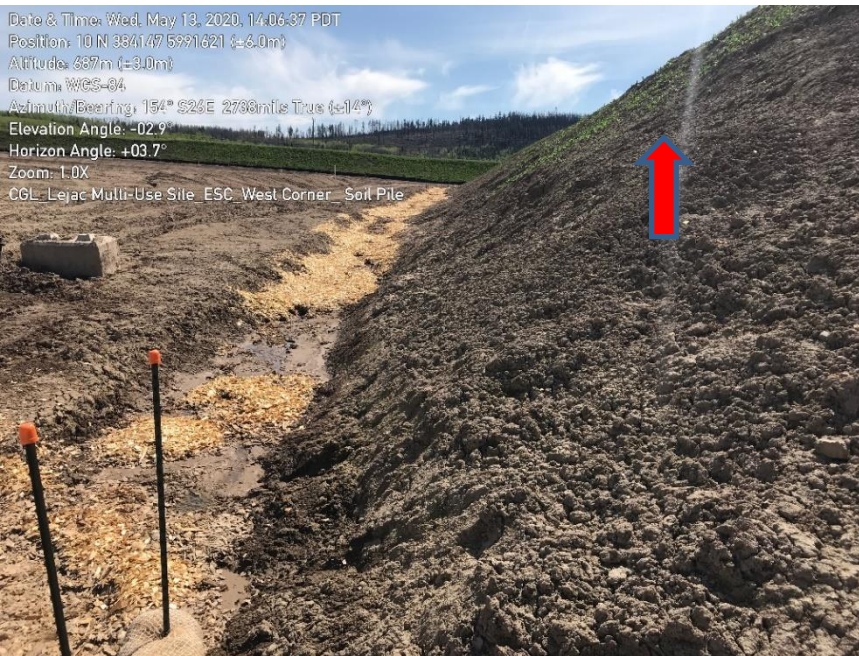
Photo 7: Soil pile with no silt fence installed along base of slope, no evidence of seeding. Vegetative growth depicted in background is weed growth associated with the seed bank within the soil pile.
