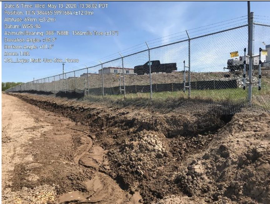
Photo 12: Northeast corner of fence line where water erosion has created a hole for animals to gain access into MUS. First identified as deficient by EAO C&E in December 2019.
