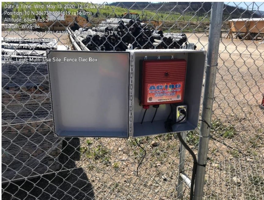
Photo 9: Electric fence energizer box – power indicator light not on.
