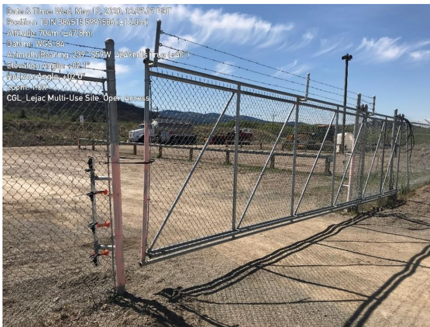
Photo 11: Main access gates depicting spacing beneath and around gate which allows access into enclosure by small wildlife.
