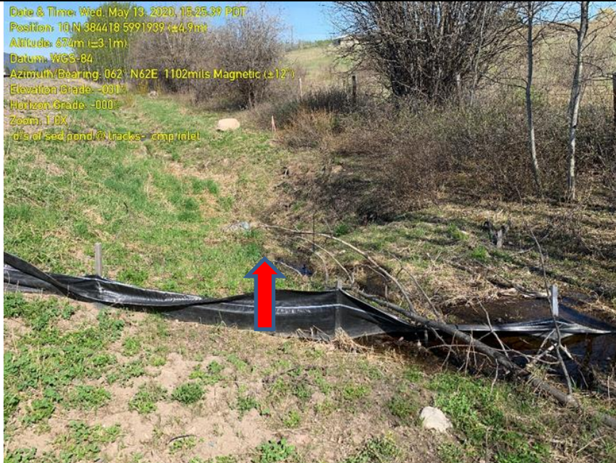
Photo 5: Culvert inlet leading beneath CN Rail tracks and directly into Fraser Lake, located within CN Rail right of way. Non-functioning ESC measures installed across the drainage.
