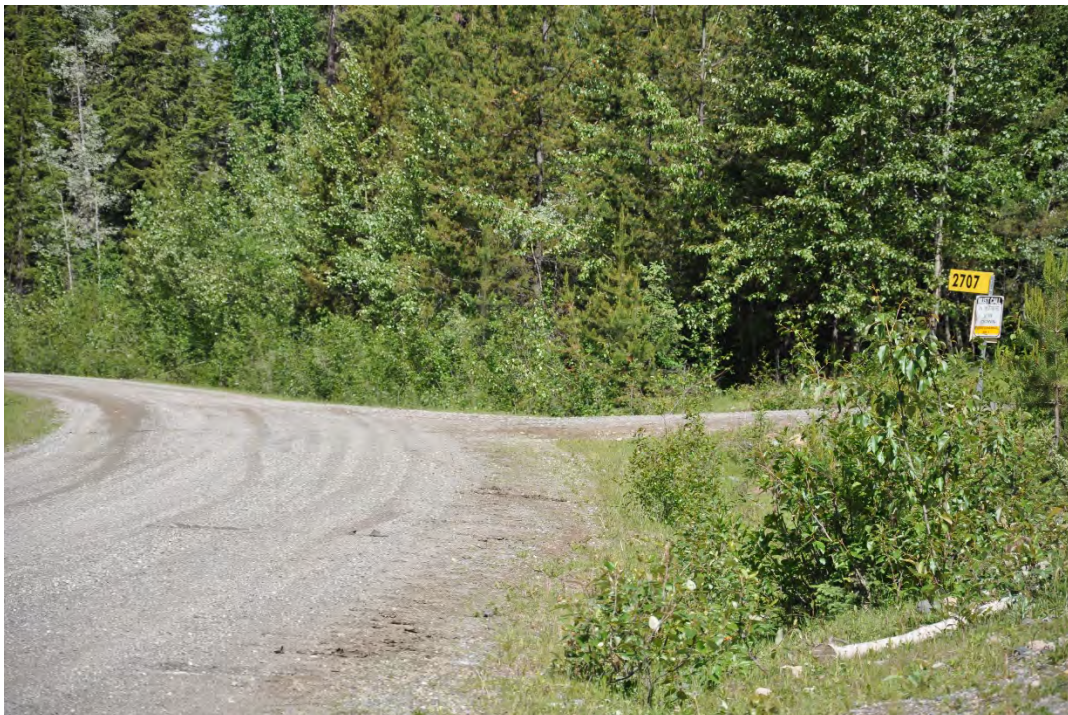
Photo 7. Typical Section of 500 Nyland Lake Road
