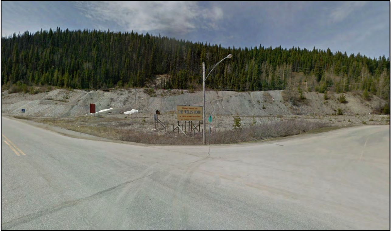
Figure 9: Current Conditions of the Island Mountain Portal Location
