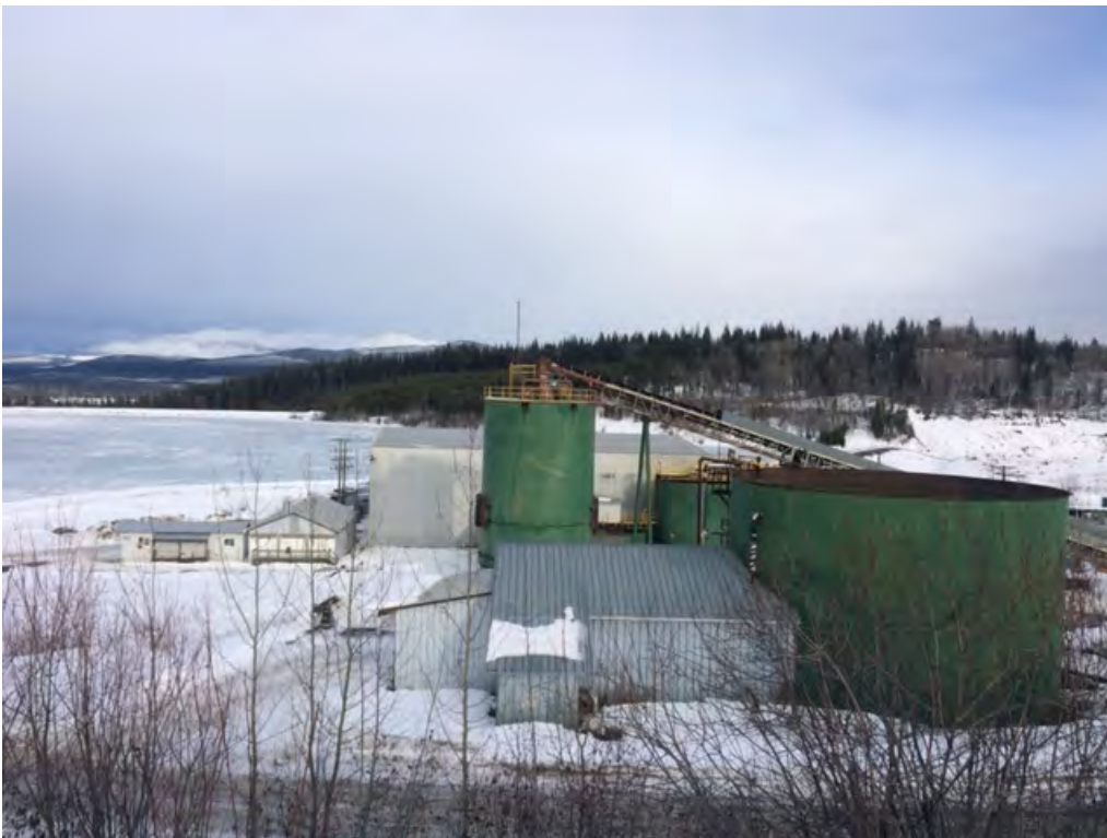
Photo 9. View of the existing QR Mill
