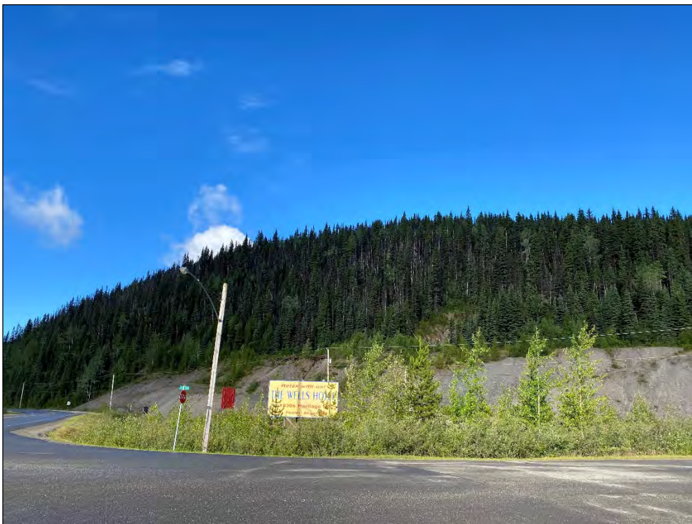
Photo 5. Island Mountain Portal Location.
