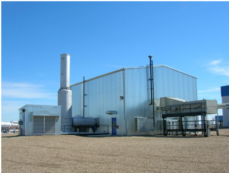
Figure 2-3: Typical compressor unit building.
