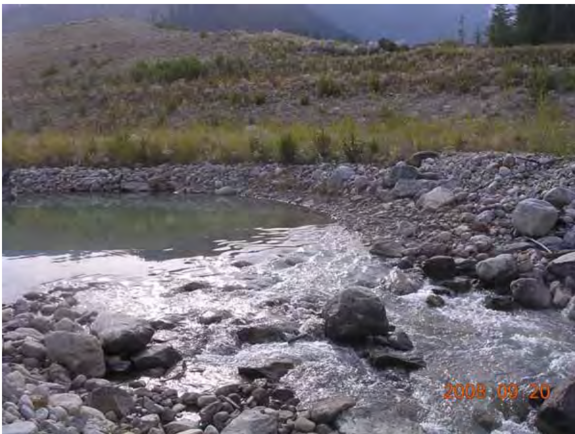
Photo 1: The outlet channel facing minor right bank scour just upstream of riffle #4.
