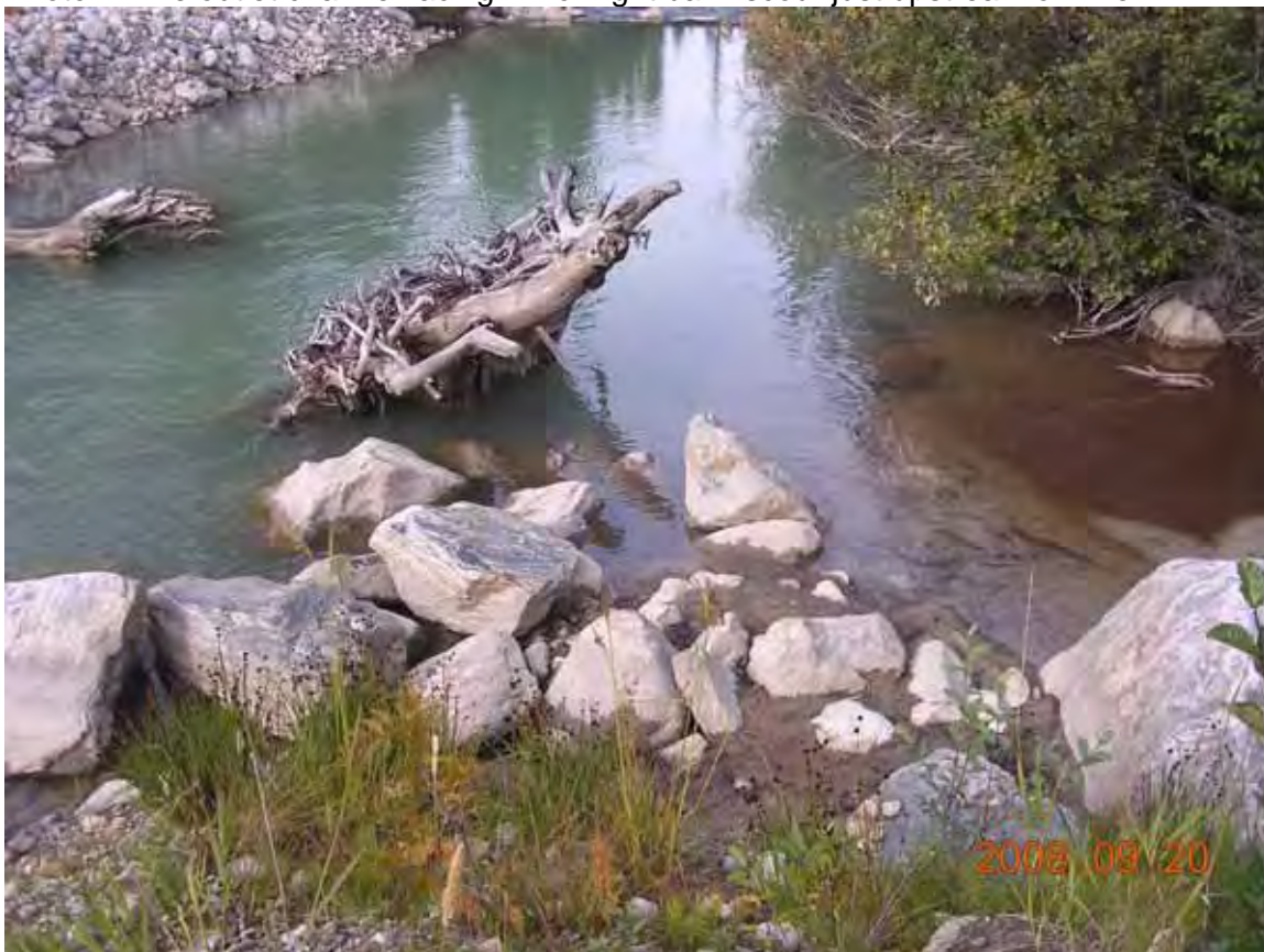
Photo 2: Stabilized right bank scour between riffle #4 and riffle #5.
