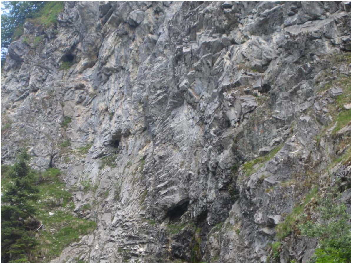
Photo 3. Karstic voids / cavities in limestone near tailings dam. June 13, 2005
