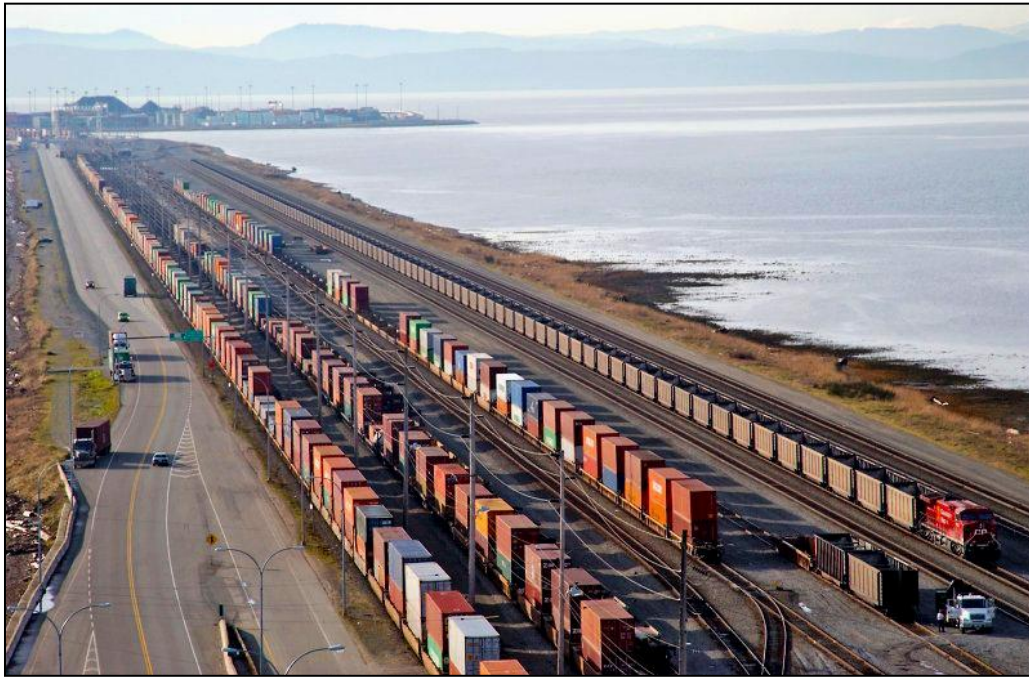
Photo 3: Existing Roberts Bank Causeway looking south, including Deltaport Way, South Yard (containers trains) and North Yard (Westshore coal trains).
