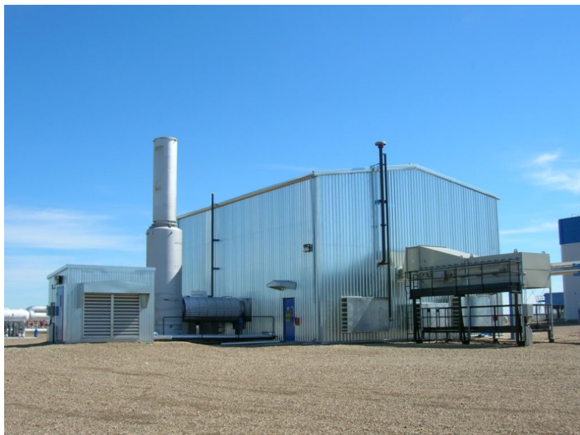
Figure 2-3: Typical Compressor Unit Building
