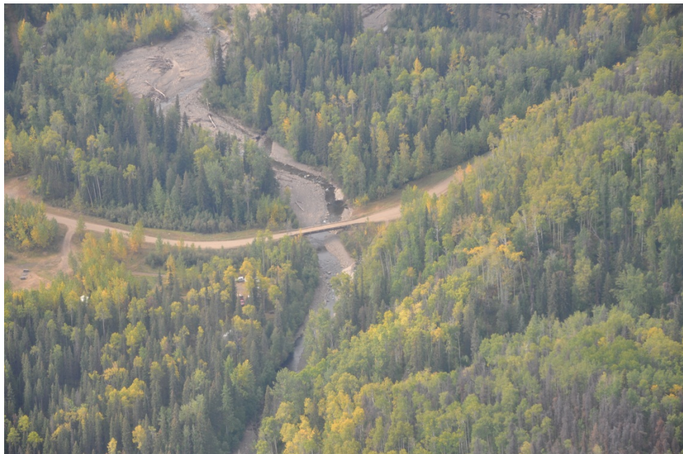
Photograph 2: Aerial view of the bridge on Johnson Creek Forest Service Road
