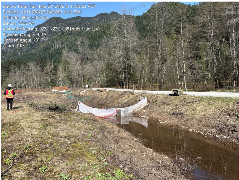
Photo 9. Fish salvage location at 8K Fishery unnamed watercourse.
