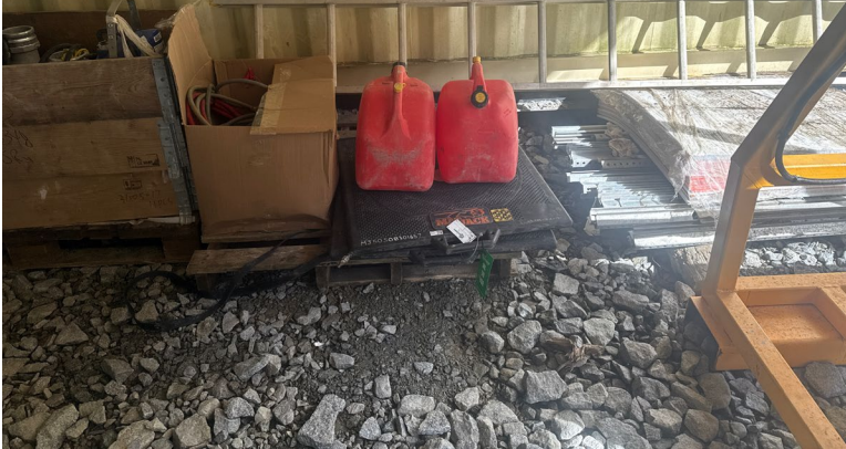
Photo 7. Fuel containers outside secondary containment.
