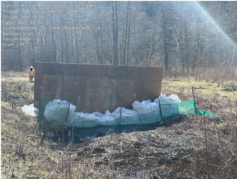
Photo 8. Watercourse isolation at 8K Fishery for fish salvage.
