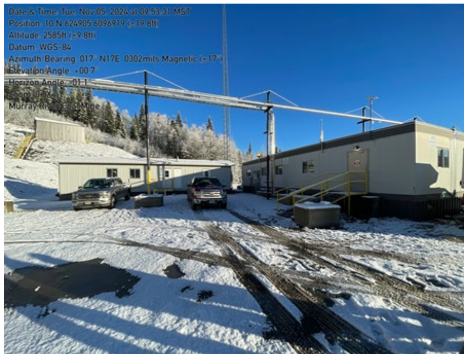
Figure 3. Modular Offices on site November 5, 2024
