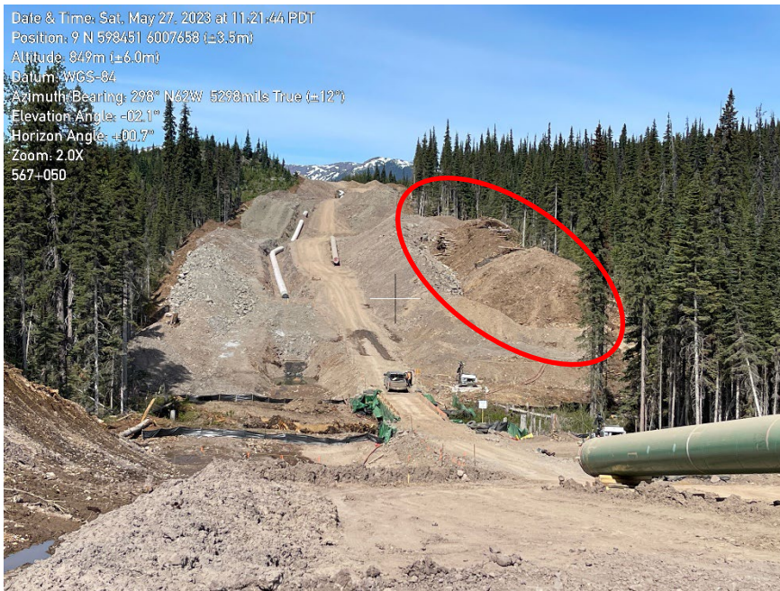
Photo 7. Soil storage at KP 567+160 to 260 not hydromulched.
