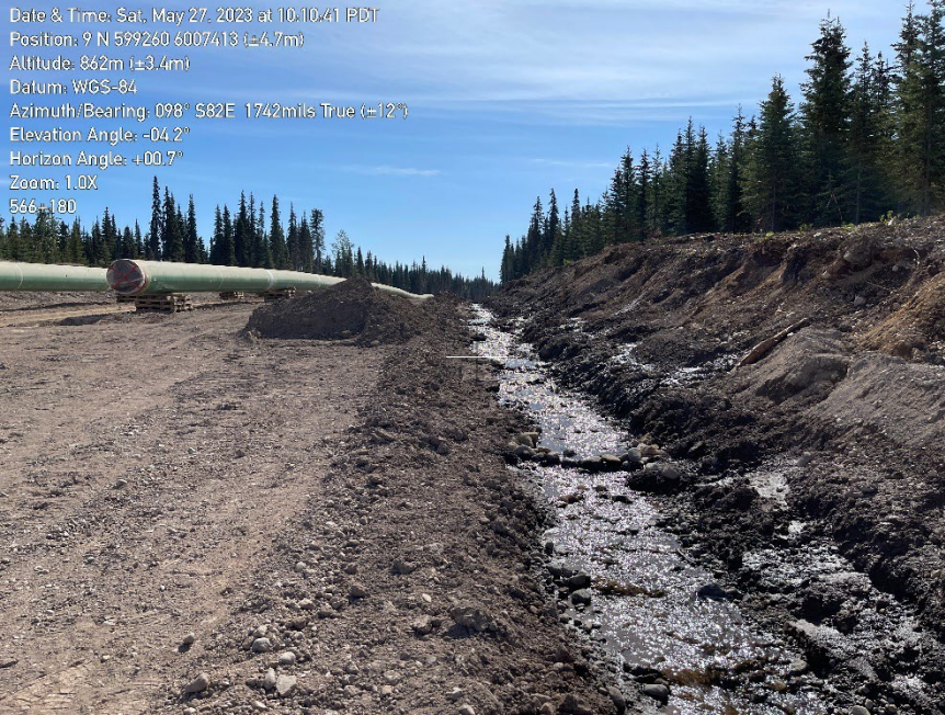
Photo 1. Unlined ditch at KP 566+180 directing NCD J430.02 to cleared wetland area.
