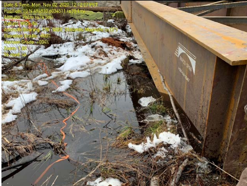
Photo 88: Steel girder in S4 channel. Left bank facing right bank.
