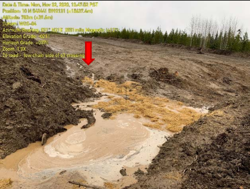
Photo 75: Sediment laden water pooling at low point of berm / water bar. Red arrow indicates erosion of exposed soils on ROW.
