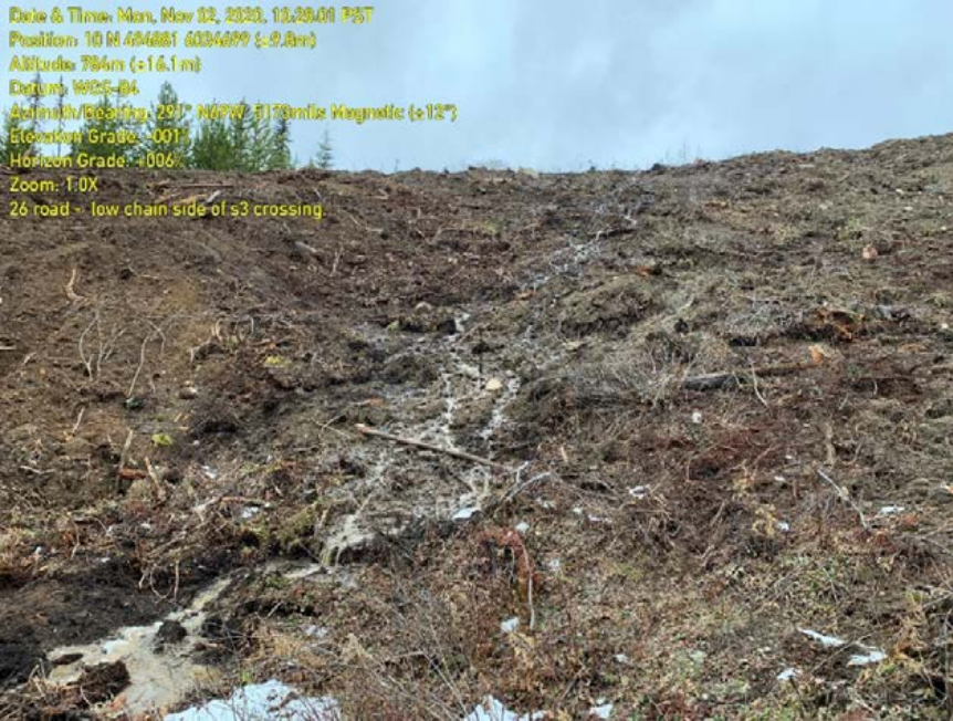
Photo 71: Exposed surface material eroding slope and draining towards fish-bearing watercourse.
