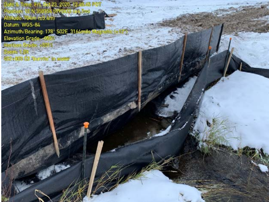
Photo 65: Geotextile within S3 channel.
