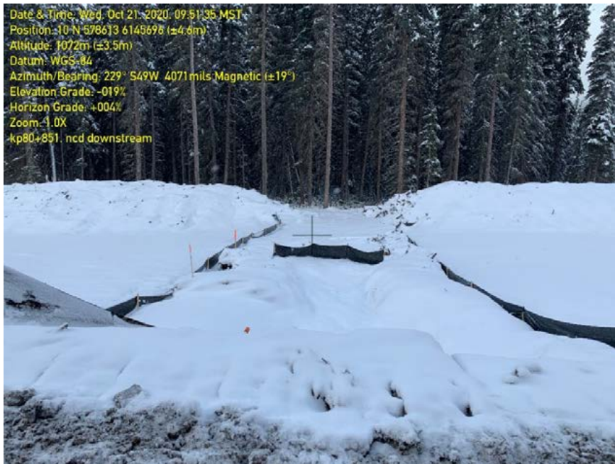
Photo 14: Sediment fence installed across an NCD feature at KP80+851.
