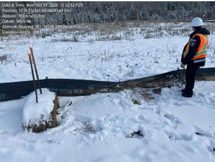
Photo 44: Work package 2. High chain looking towards low chain at Crooked River DPI. Large exposed area and soil stockpile all flows to this section of sediment fence. Fence overwhelmed and had previously failed.
