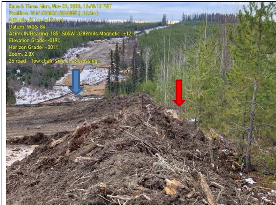
Photo 79: Red arrow indicating sediment laden water on back side of windrow continuing to flow down slope. Blue arrow indicates fish-bearing stream at base of slope.
