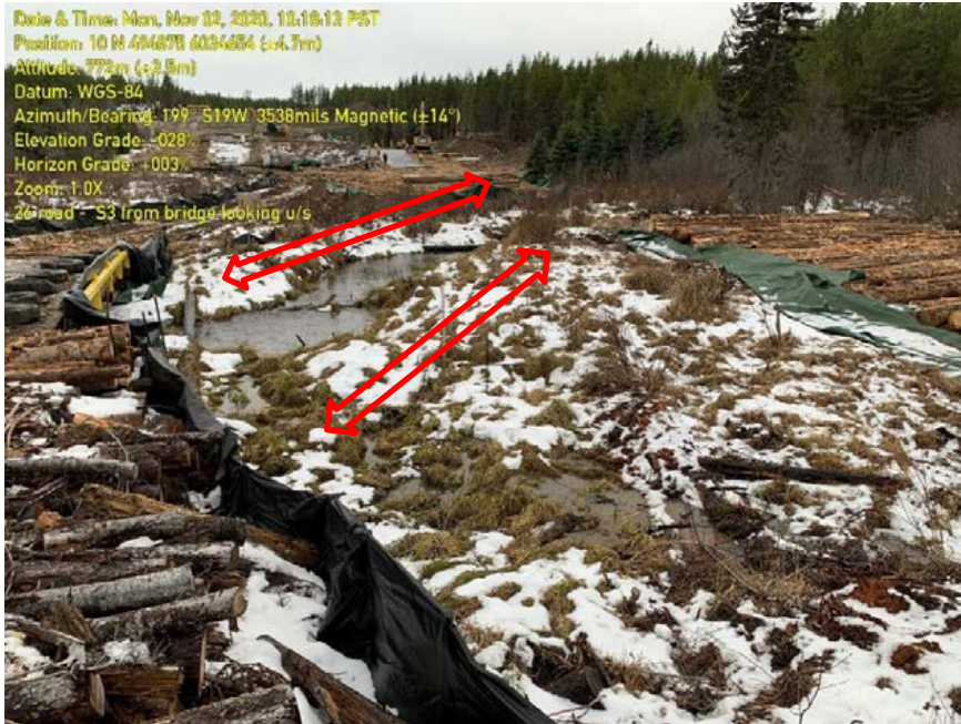
Photo 66: KP 244+510, low chain looking towards high chain. No ESC measures along banks of S3.
