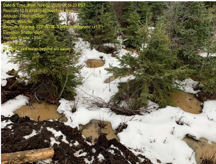
Photo 85: Sediment laden water in vegetation beyond water bar discharge location. Risk of this material reaching S4 feature.
