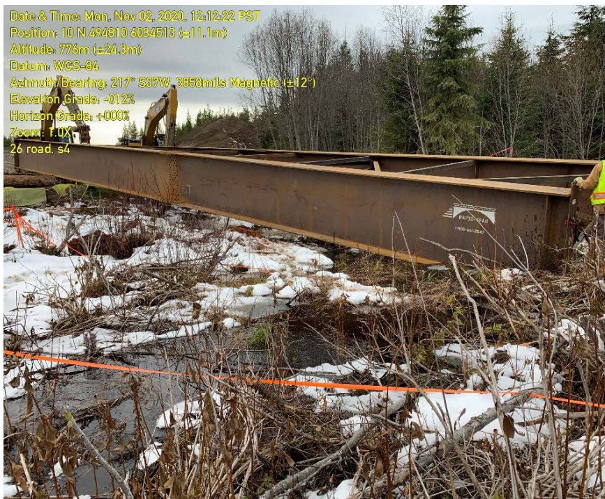
Photo 89: Steel girder in S4 channel. Downstream facing upstream.
