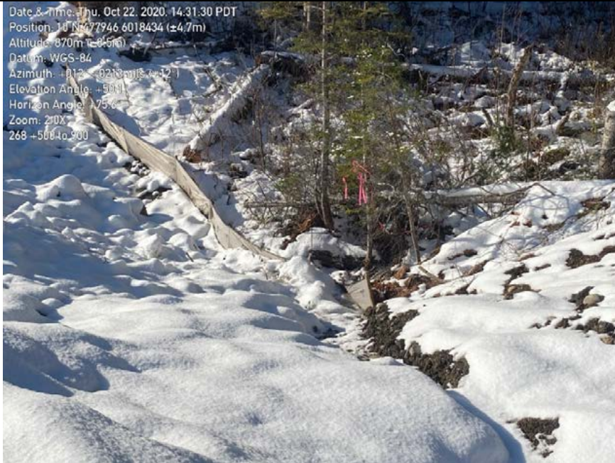
Photo 27: Sediment fence overwhelmed and at risk of failing, signs of gully erosion can be seen leading toward this section of the fence. NCD at base of slope.
