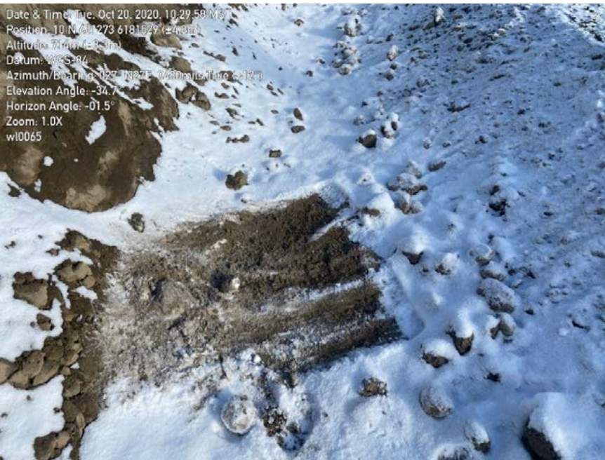
Photo 5: Fine soils in ditch line from photo above.
