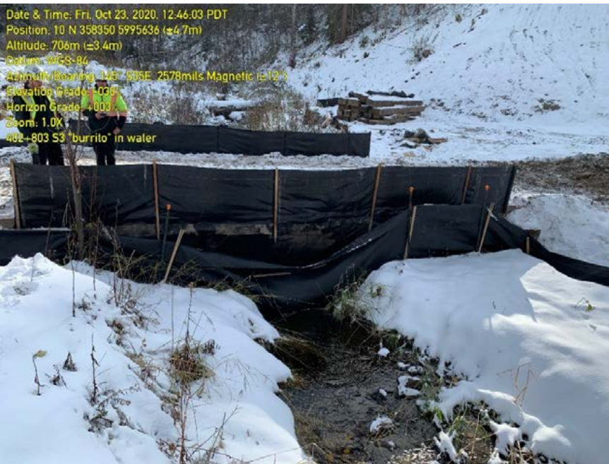
Photo 64: Work package 3. Geotextile beneath bridge containing sediment and sagging into the water of fish-bearing (S3) watercourse.
