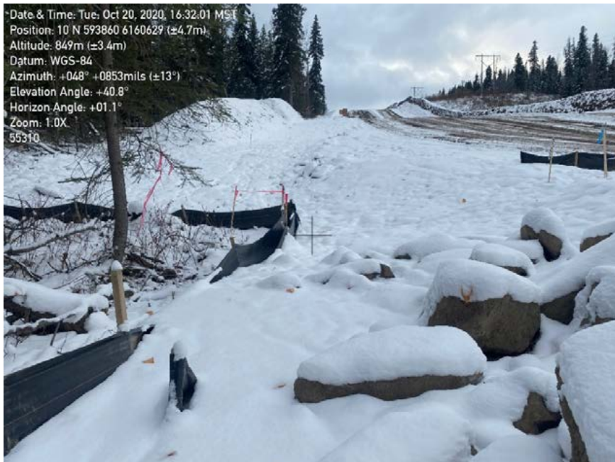
Photo 36: Work package 1, KP55+310. Material from ROW eroded and transported to this section of sediment fence. Sediment fence overwhelmed.
