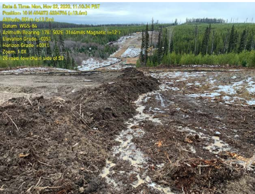
Photo 70. Water from water bar directed to back side of berm and flowing towards watercourse. Erosion taking place and sediment mobilizing towards watercourse #WC272.
