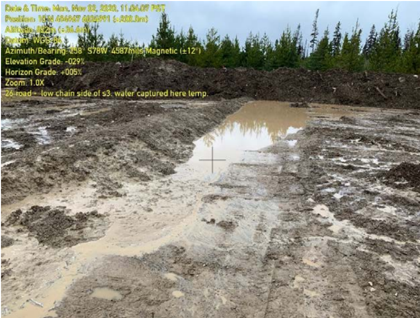
Photo 72: Berm used to direct water from ROW to low point.
