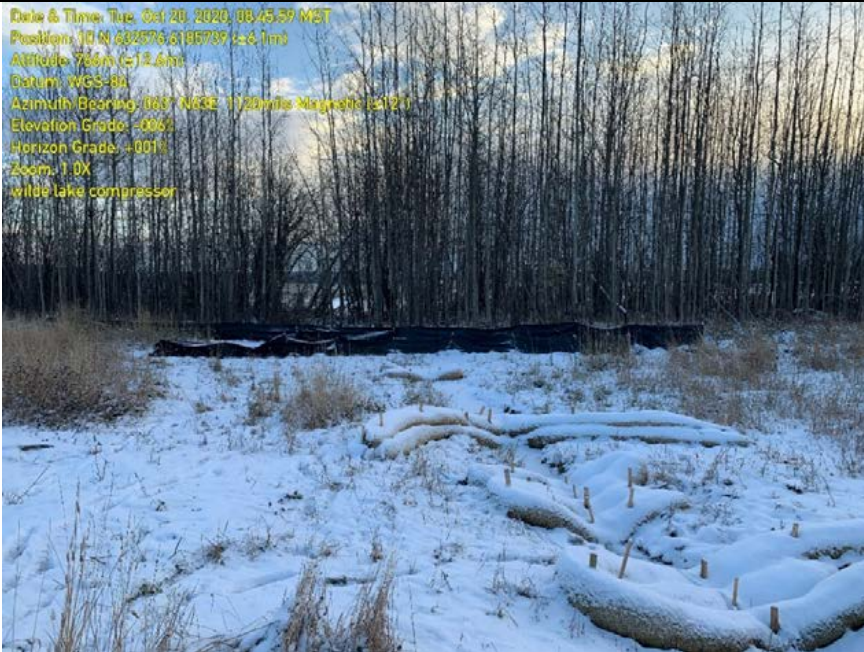
Photo 15: Sediment fence across outlet channel at Wilde Lake Compressor Site.
