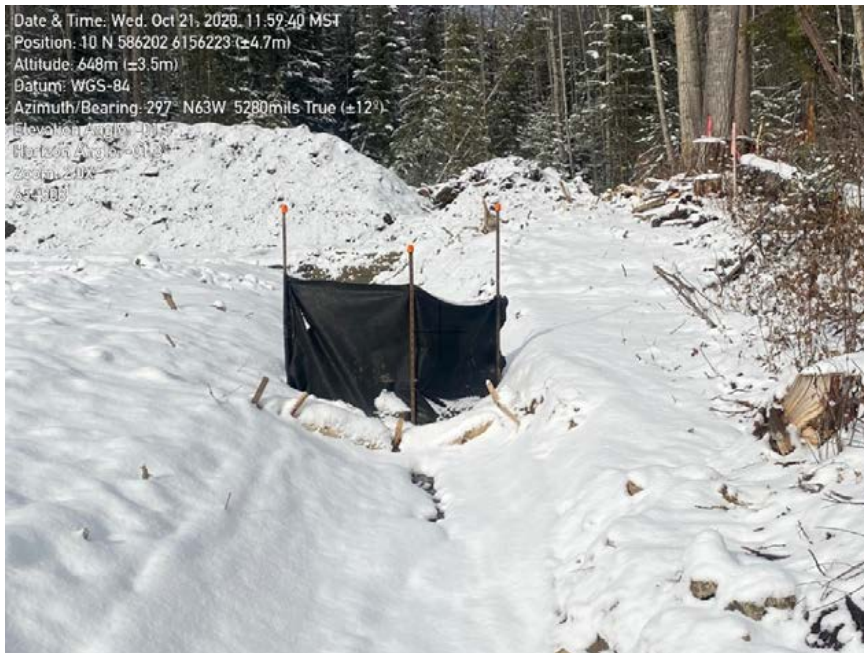
Photo 20: Example of sediment fence installed across a ditch.
