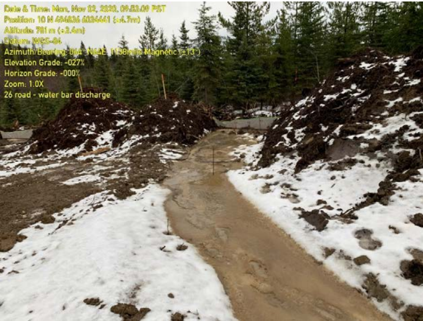
Photo 83: Water discharge location from lower most water bars.
