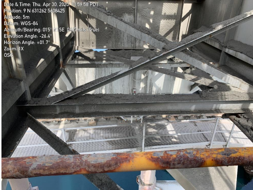
Photo 4: Piled material on cross beams under convayor belt on shiploader.
