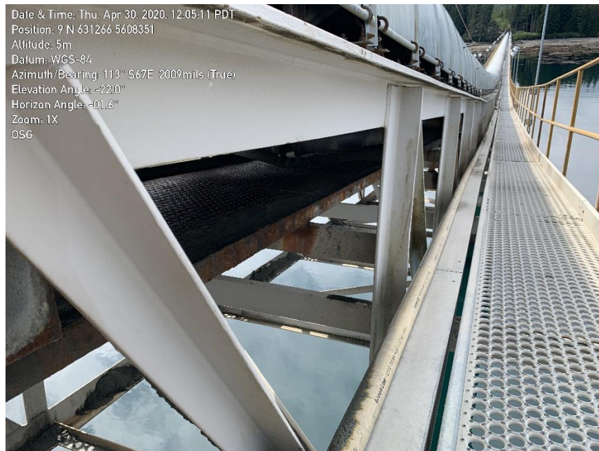
Photo 1: Newly constructed spill tray from shoreline to ship loader.
