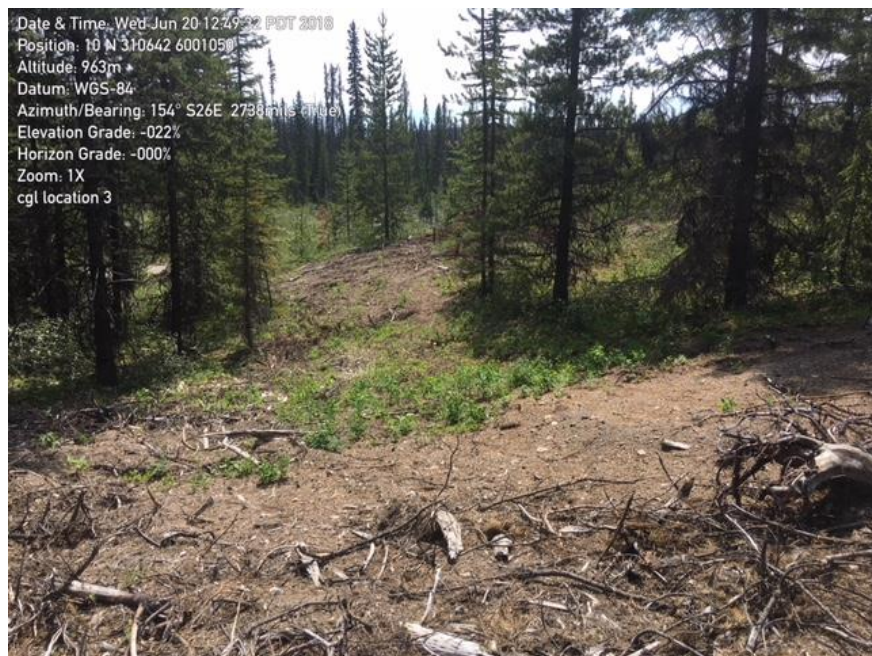
Photo 1: Vegetation clearing and ground disturbance at “West of Anders Lake 10U 310588E, 6000988N”, CGL descriptor “Borrow Site PBS52”.
