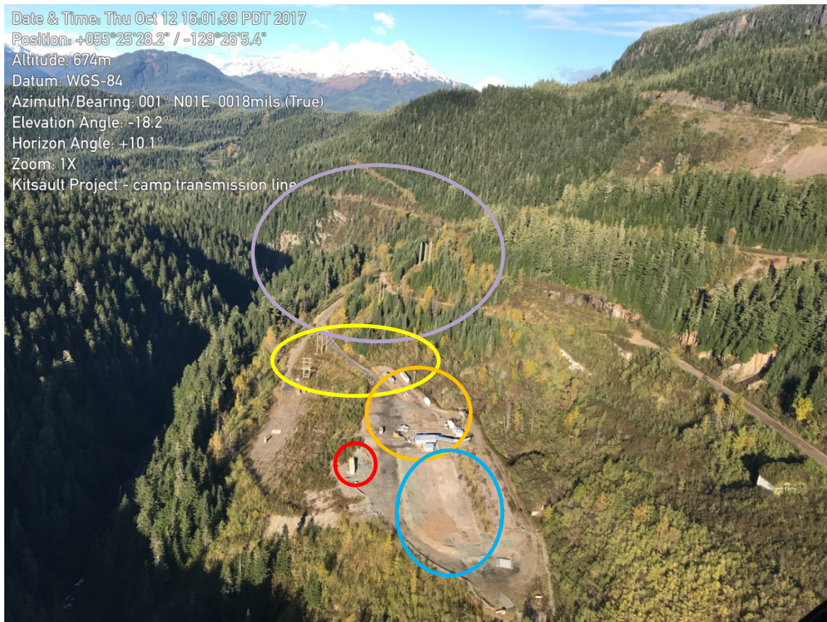
Figure 7: Exploration camp (orange circle) at the historic Clary Dump site, looking south. Transmission line terminates at the exploration camp (yellow circle). Vacant pad (location of temporary construction camp, blue circle). Wastewater/Sewage treatment plant southeast of camp (red circle). Proposed Low Grade Stockpile (LGS) area (purple circle).
