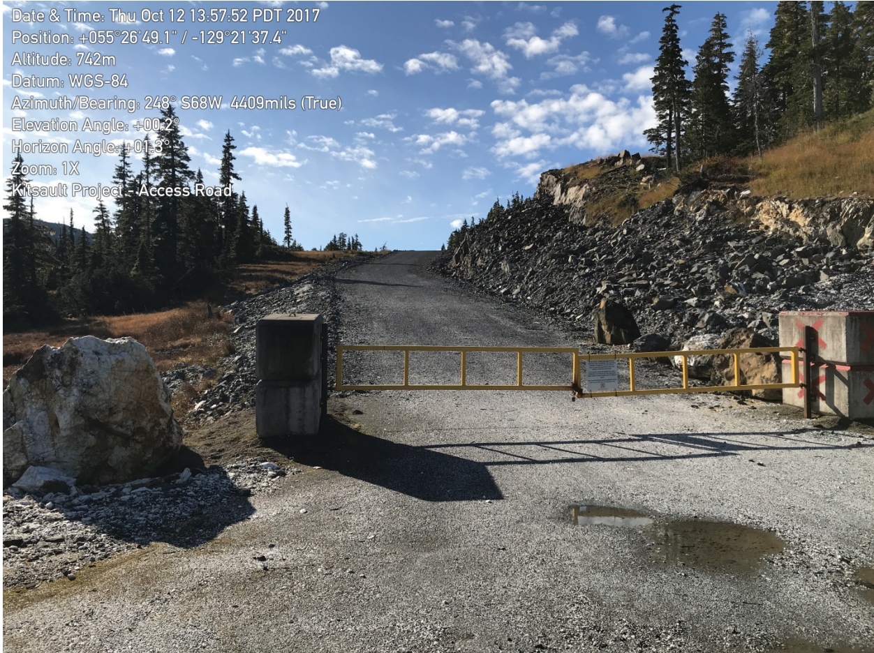
Figure 3: Mine Gate, on the access road to the Plant Site Area. Access road constructed to accommodate two way light vehicle traffic to and from main Mine site area and concentrate haulage from the process plant to market.
