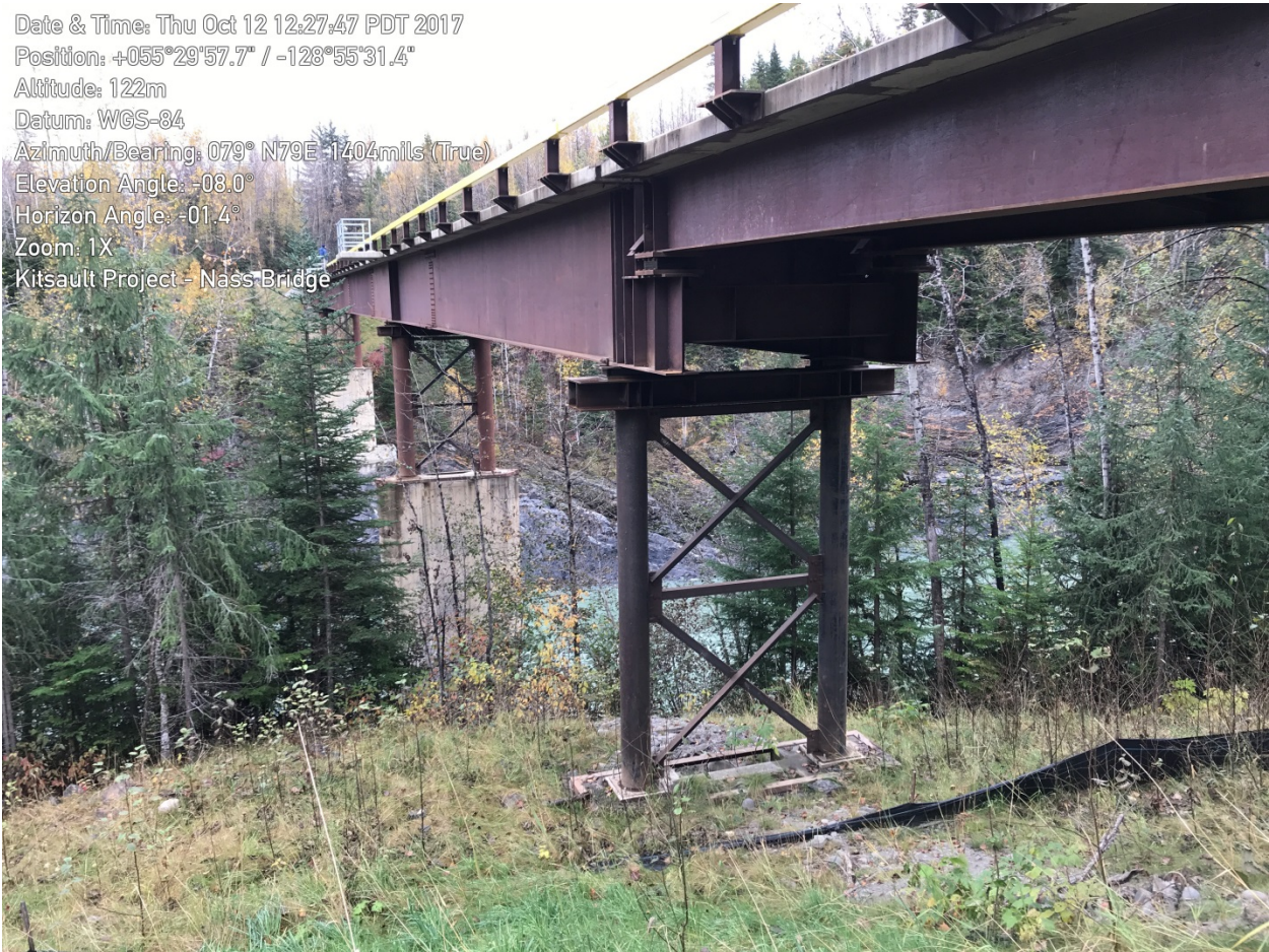
Figure 8: Nass Bridge, looking east. Vegetation and silt fence in foreground.
