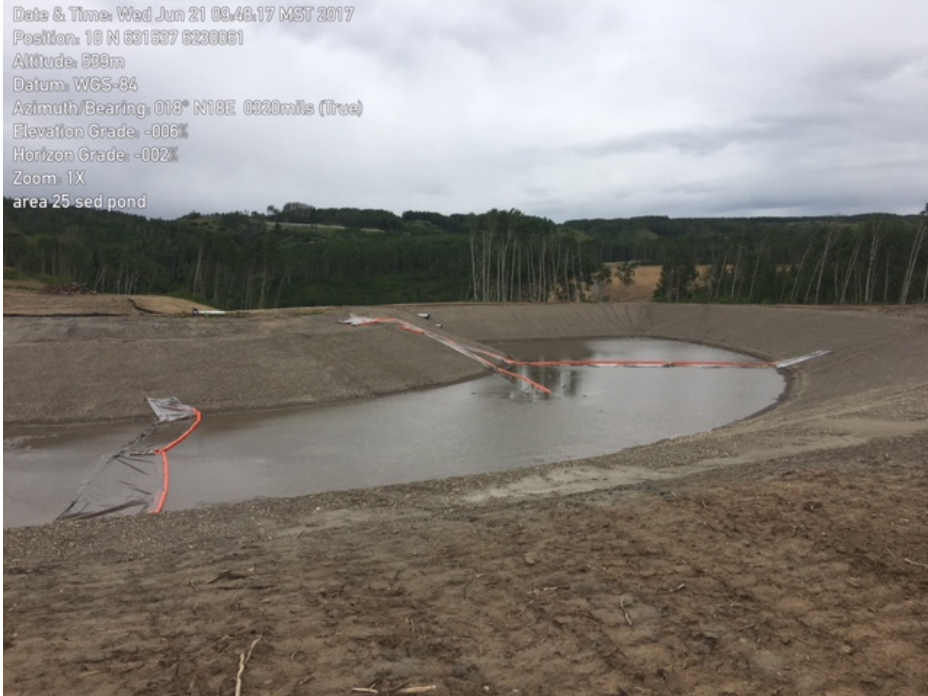
Photo 2: Area 25 sediment pond. Note sediment curtains.
