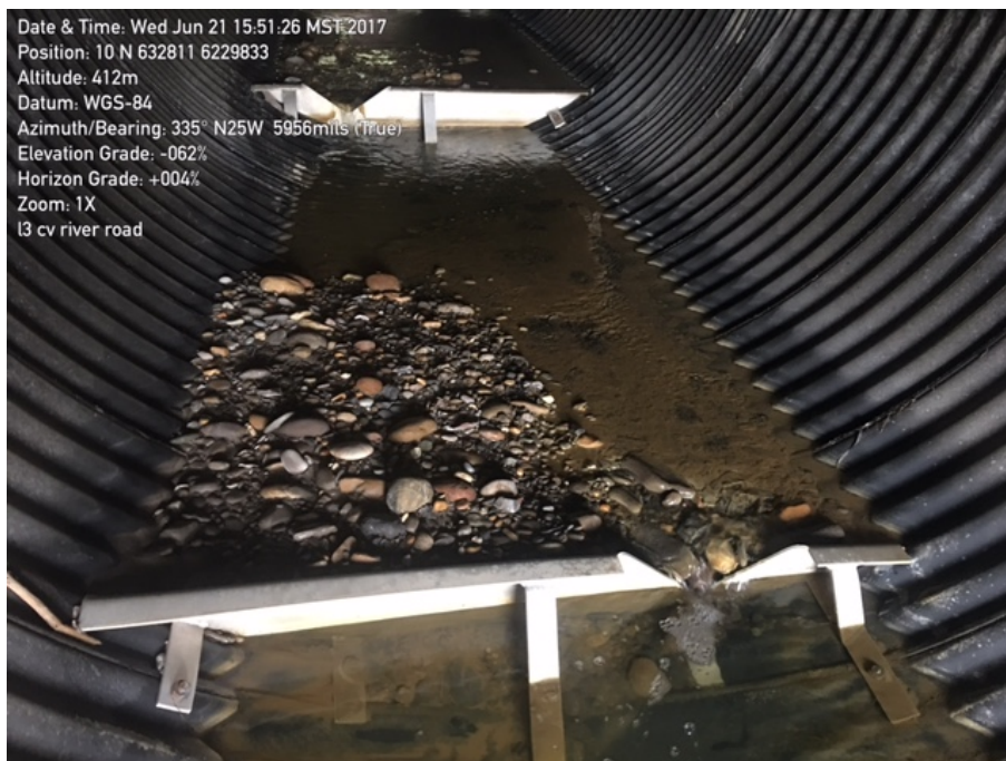
Photo 8: L3 culvert under River Road. Note culvert baffles filled with coarse sediment
