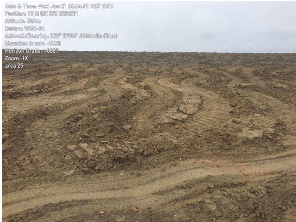
Photo 1: Example of surface roughening implemented in Area 25 and the upper L3 watershed.
