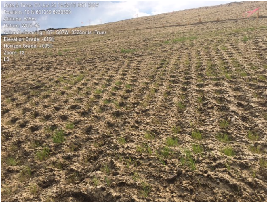
Photo 3: Hydroseeding and surface treatment implemented to reduce erosion and sediment transport, top of bank, L3 ravine.
