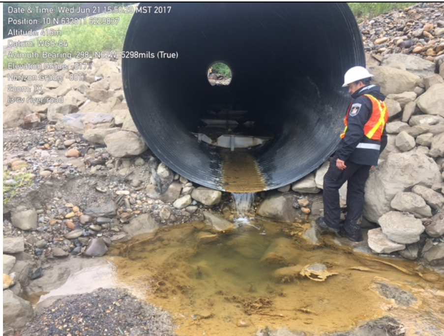
Photo 7: Culver under River Road at the L3 watercourse. Looking upstream from downstream end. Note downstream end of culvert is perched and limited plunge pool depth.
