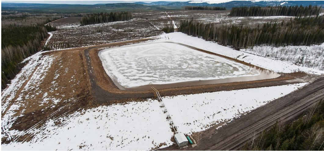
An unauthorized Progress Energy dam where millions of gallons of freshwater was found impounded in early April. It is among "dozens" of unpermitted dams spread across northern B.C. Photo © Garth Lenz, all rights reserved.
