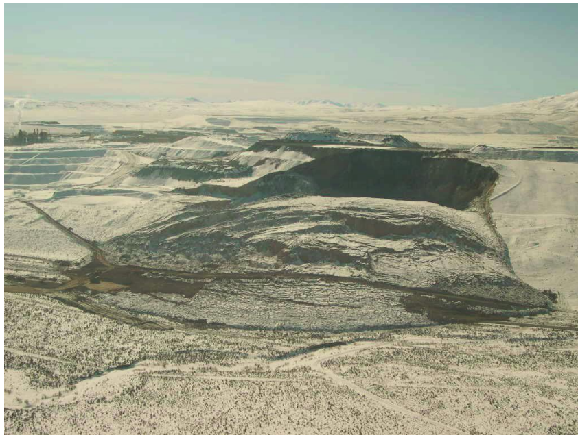
Waste Rock Failure, Gold Quarry Mine, Nevada, February 5, 2005
