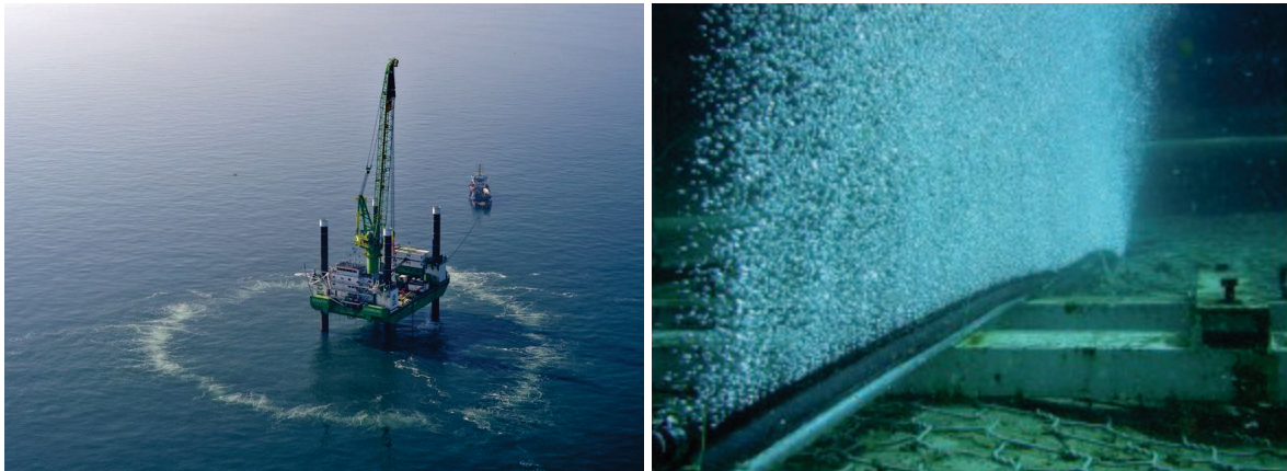
Figure 2. Example of air bubble curtain. (Left): Active air bubble curtain around pile driving activities. (Right): Tubing for an active air bubble curtain.
