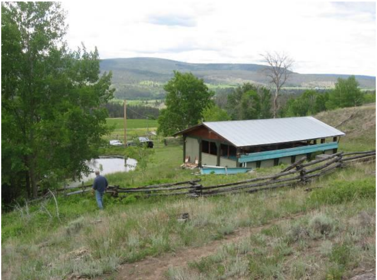
Figure 8-14 Hatchery NE View
